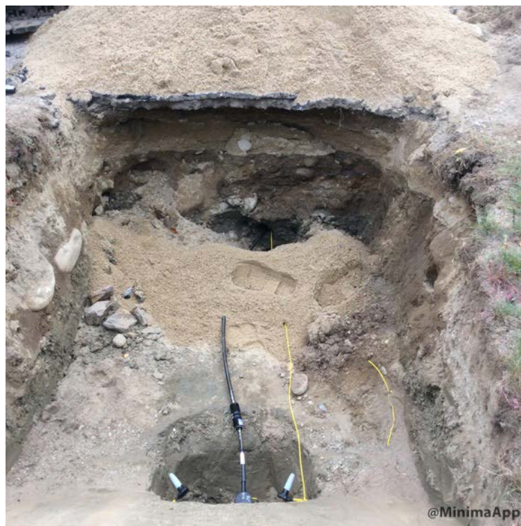
Undermining of Meadow Lane for gas service
