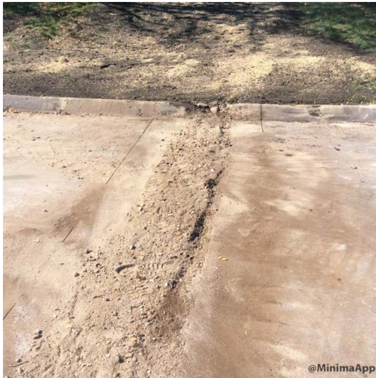
Backfill compacted and I' cutbacks.
