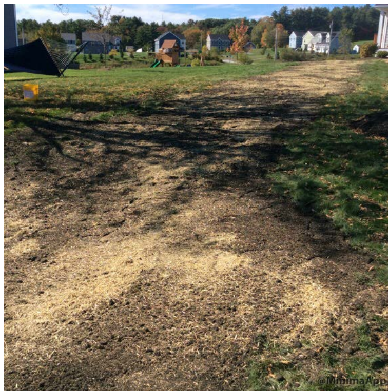
Loam, seed, and mulch placed in the disturbed vegetated area.
