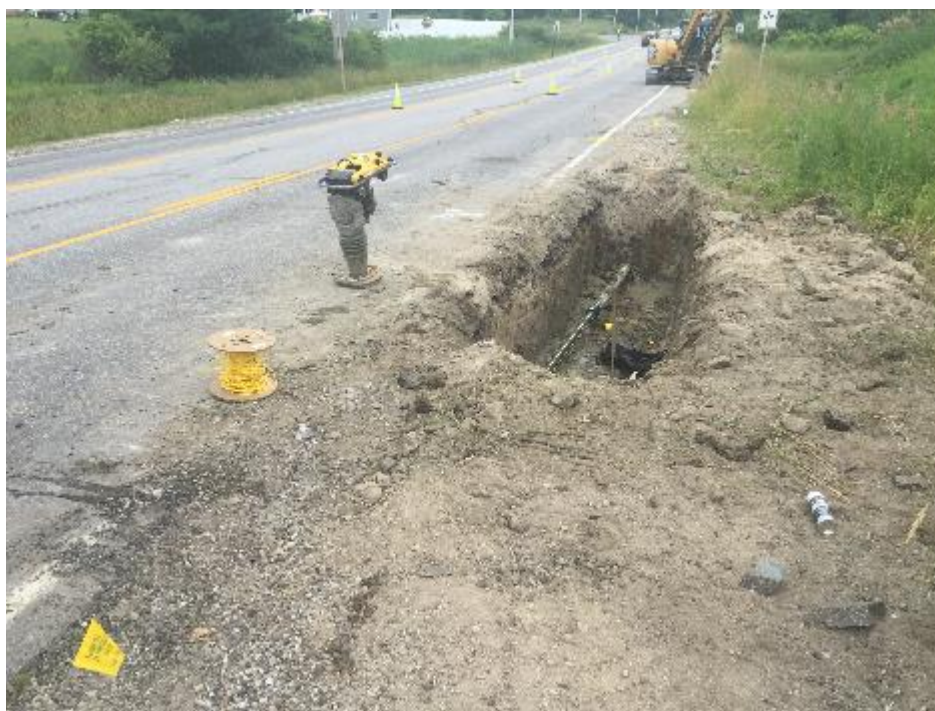
Trench and compactor awaiting backfill off Route 100
