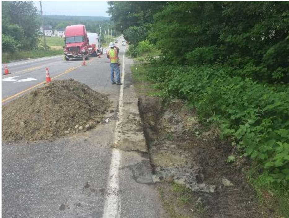
Trench excavated off roadway of Route 100
