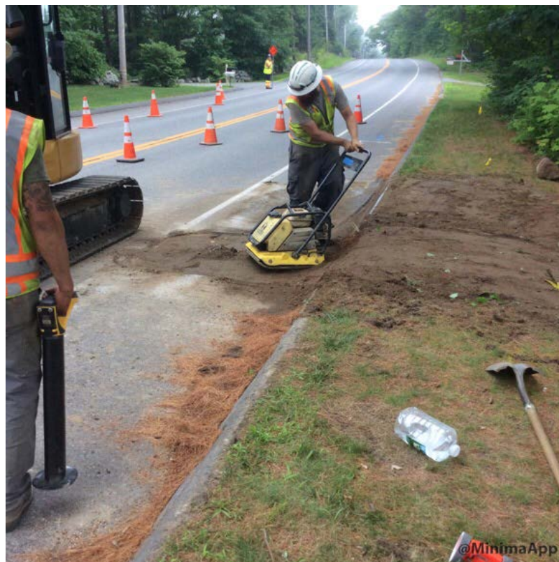
Compacting gravel backfill
