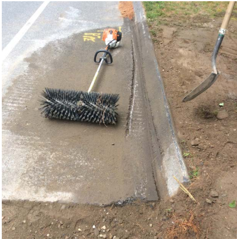
Scratch from excavator bucket
