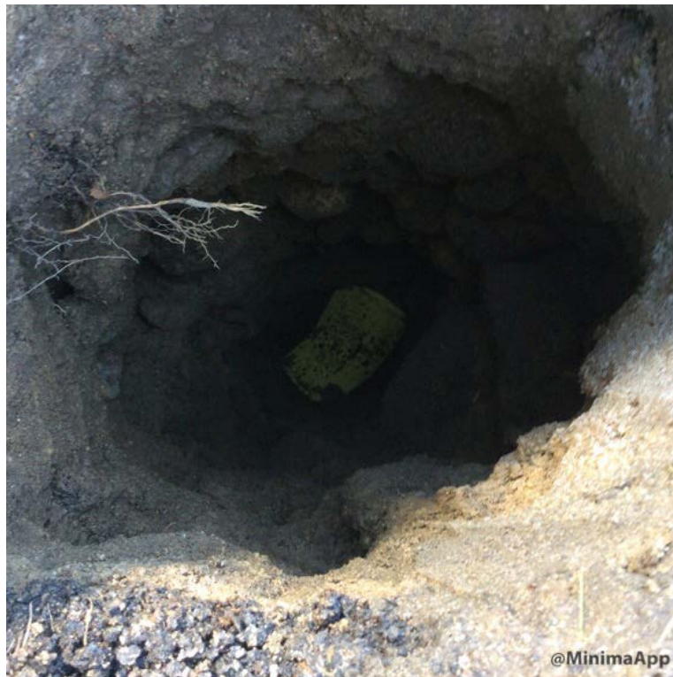
Rock shield placed over water service.
