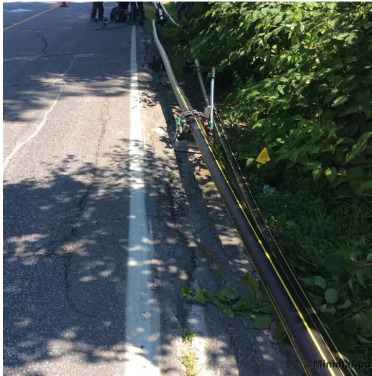
Fusing pipe on Route 100.
