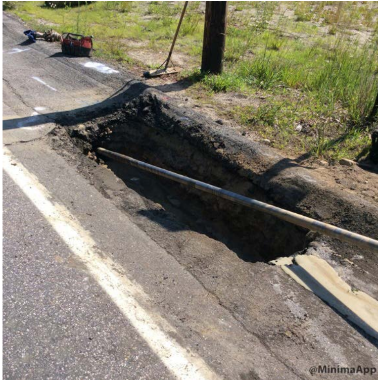
Excavated shoulder trench for directional drill method.
