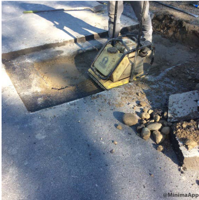
Compacting gravel with plate wacker.
