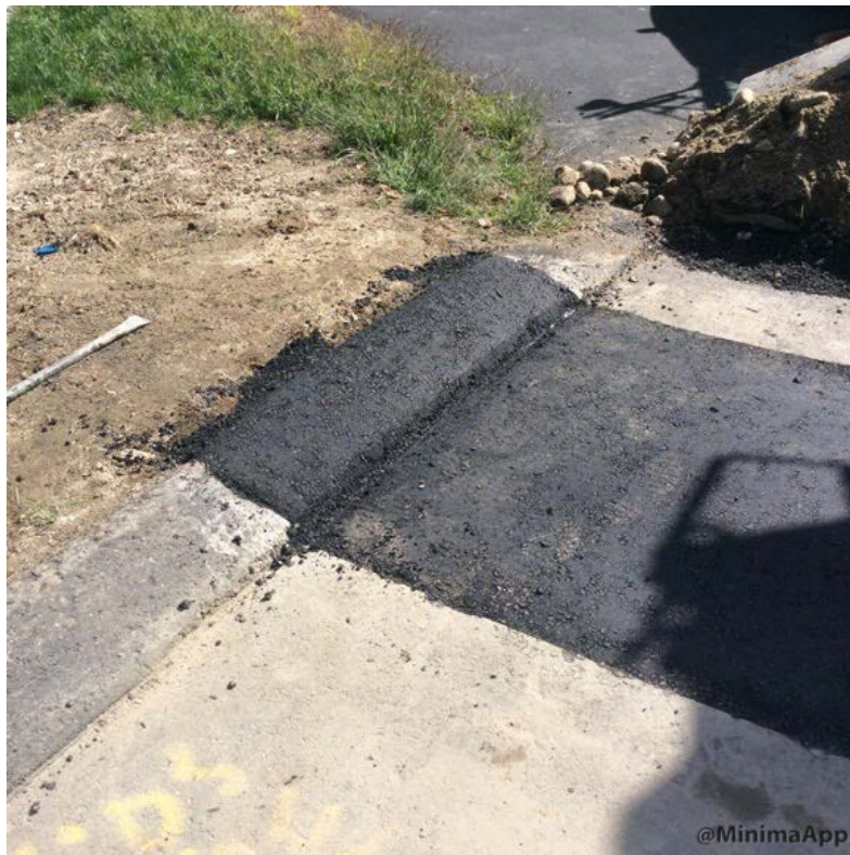
Completed trench paving with hand built curb.
