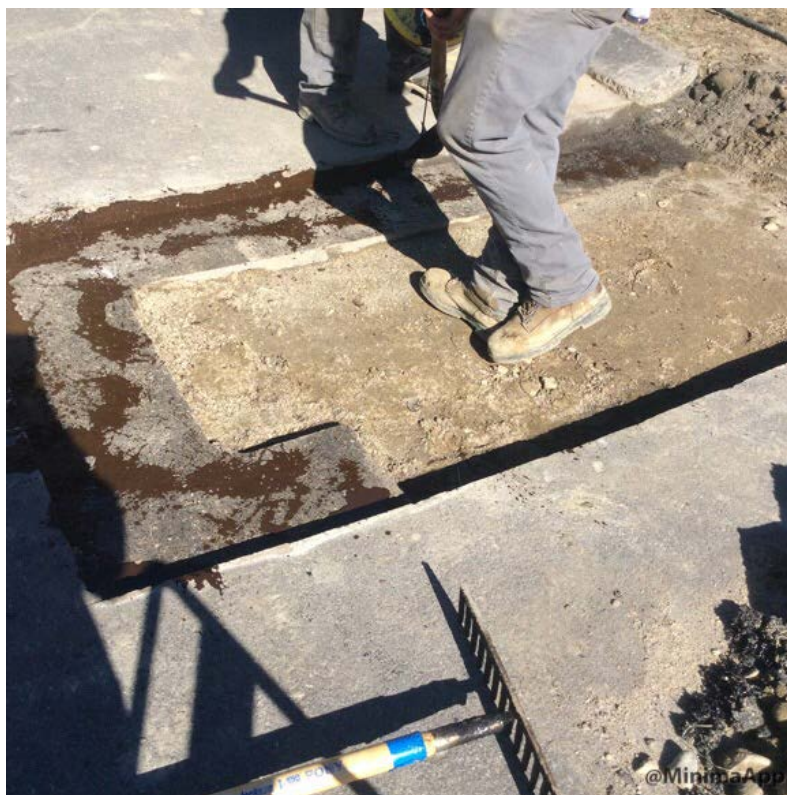
Tacking existing pavement.
