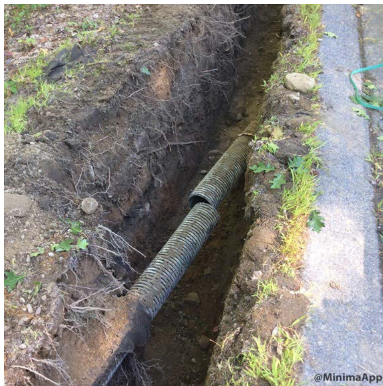
Sawcut underdrain prior to pipe install and repair.
