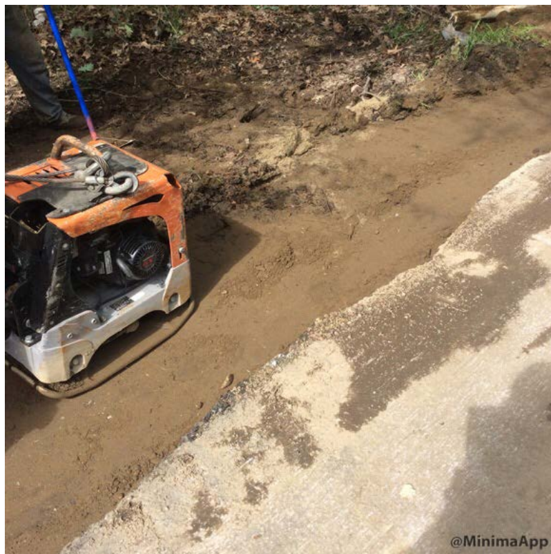
Compacting backfill with plate wacker.
