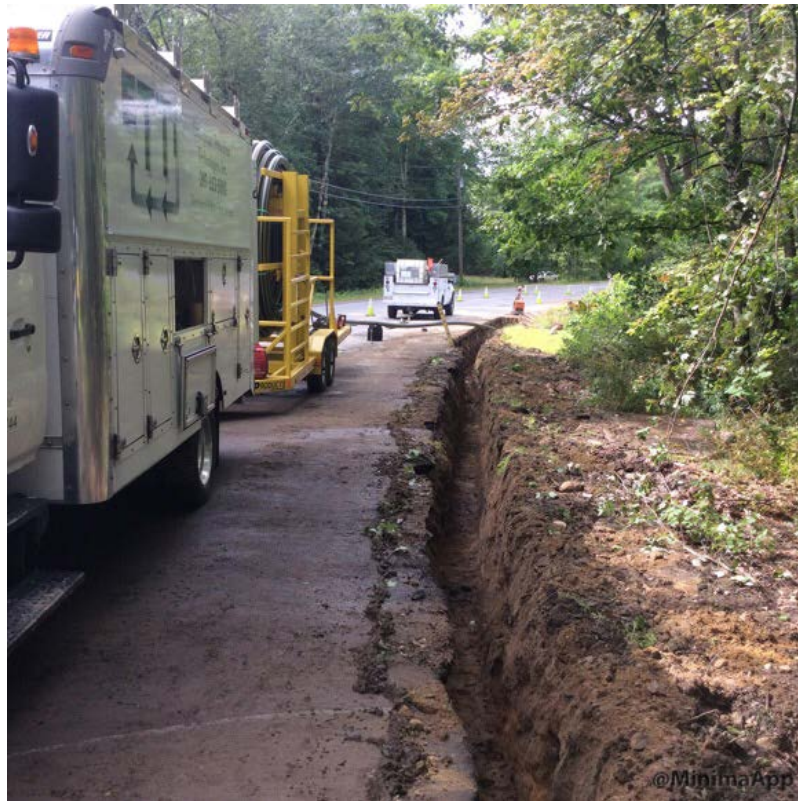
Preparing to install pipe in open trench.
