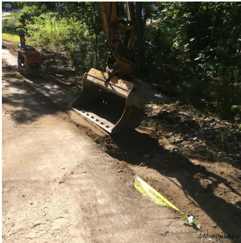
Placing backfill with excavator.
