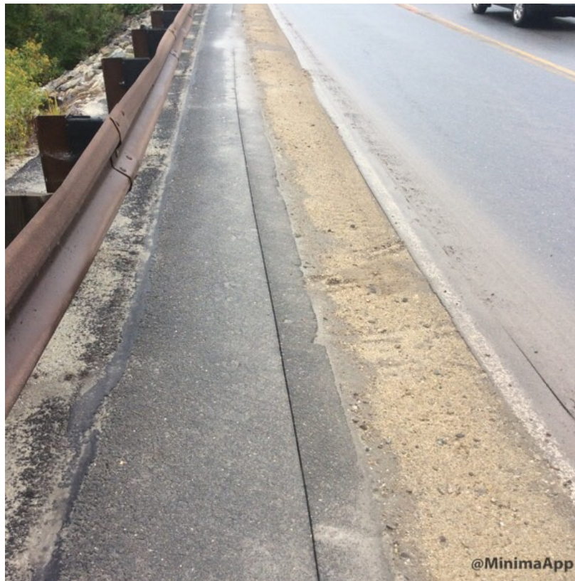
Crew sawcut pavement near large culvert
