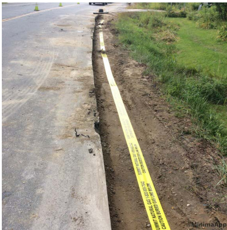
Backfill compacted and warning tape placed in gas main trench.
