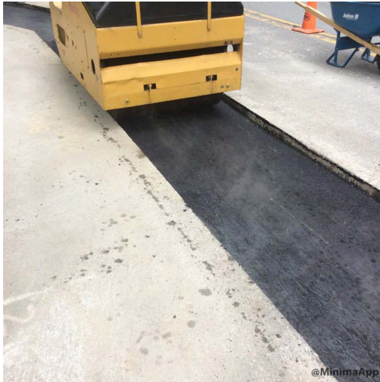
Compacting the first lift of 12.5mm HMA with 3 ton vibratory roller.
