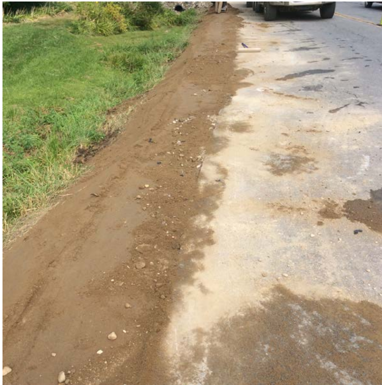
Final lift of backfill compacted.
