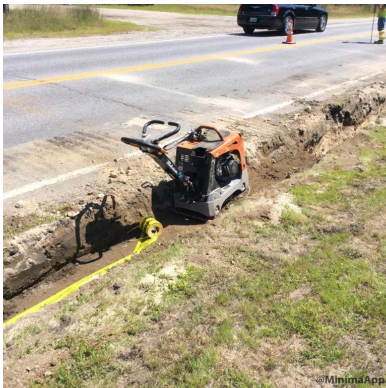
Compacting backfill in front of D.J. Small
