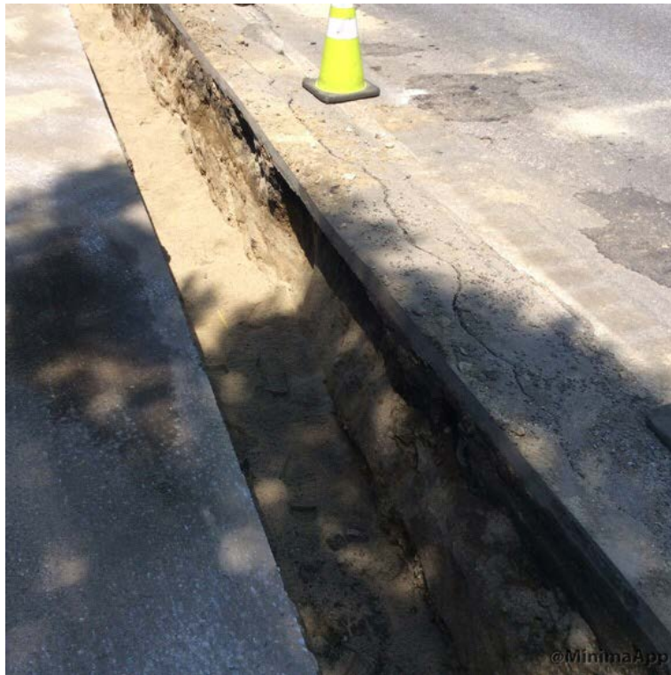
Undermining at driveway crossing trench
