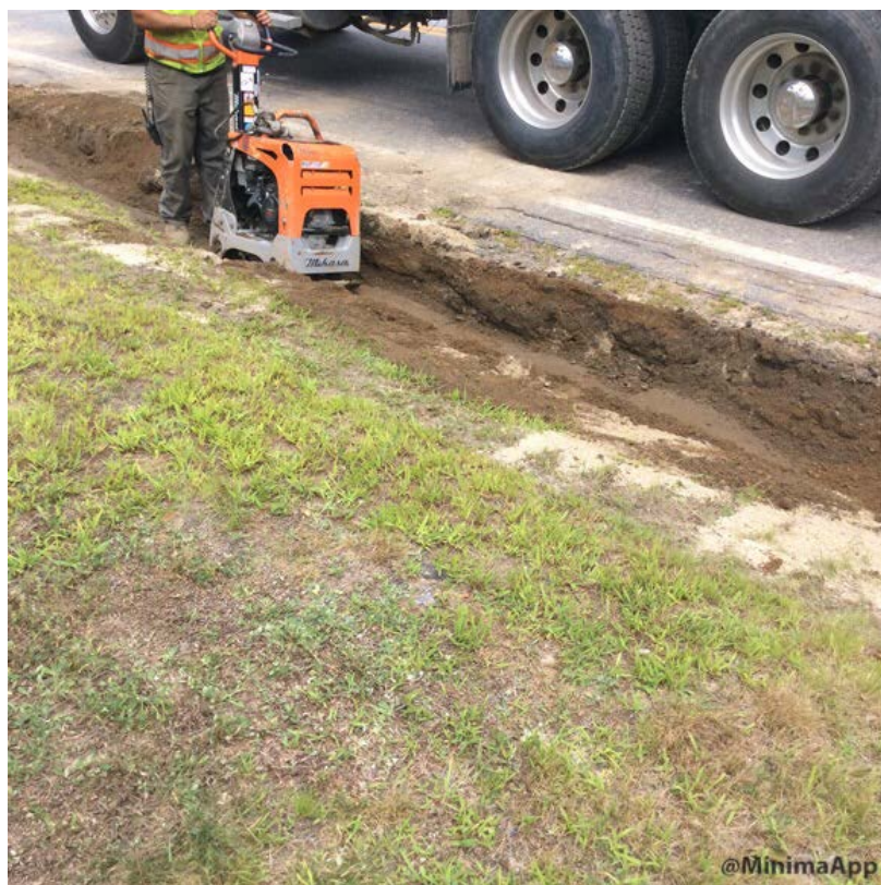
Compacting backfill with plate wacker
