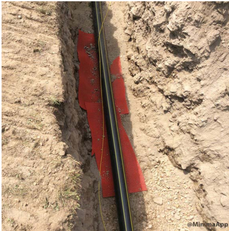
Rock shield placed at stormdrain crossing
