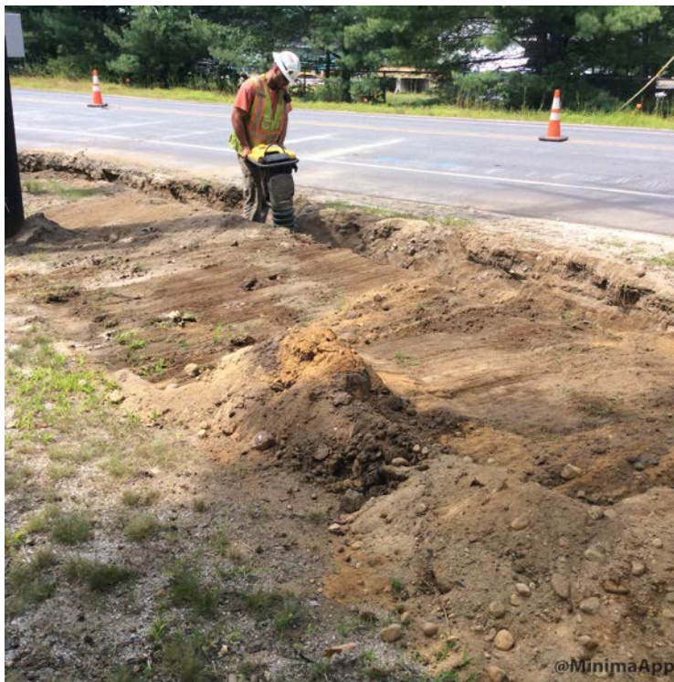
Compacting backfill with jumping jack
