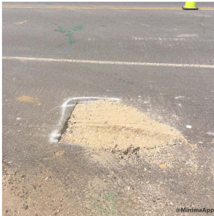
Pothole at seam of Blackstrap Road and West Cumberland Fire Station driveway
