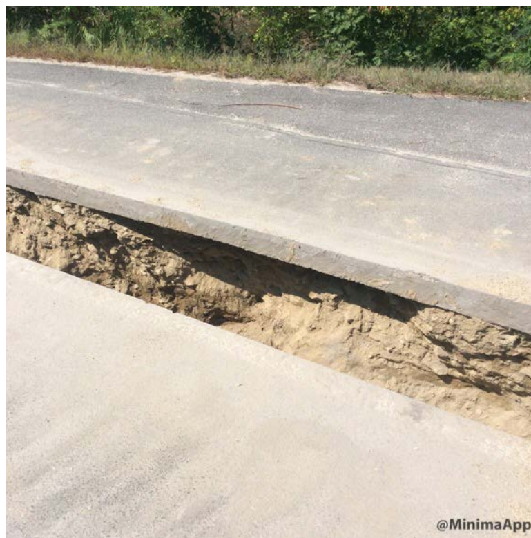
Pavement undermined on western side of large culvert.
