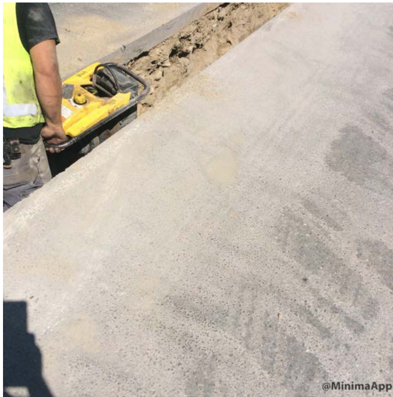
Compacting sand layer with jumping jack
