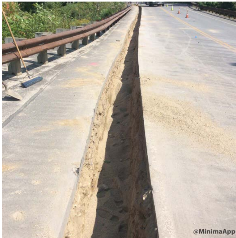
Open trench over large culvert.
