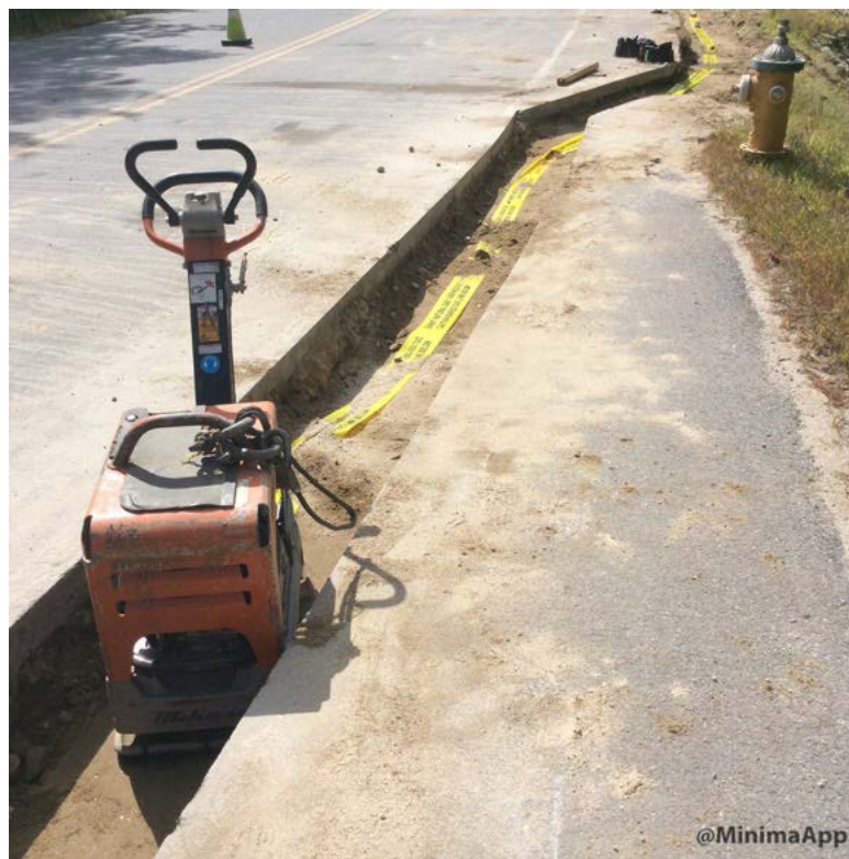
Backfill compacted with plate wacker and warning tape placed.
