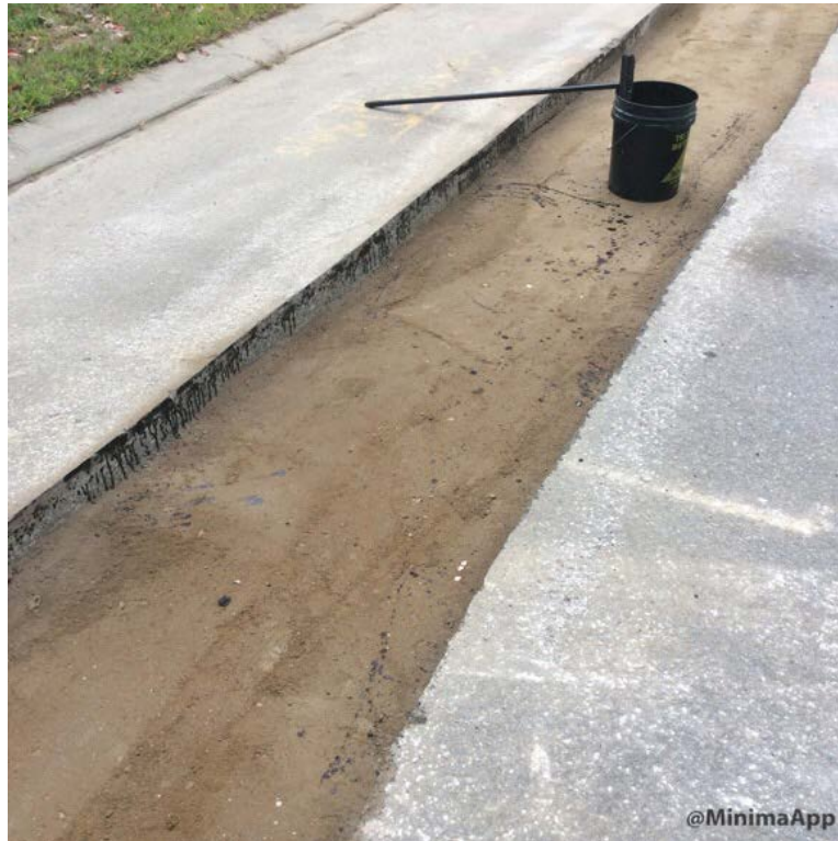
Gravel compacted and edges of pavement cleaned and tacked.
