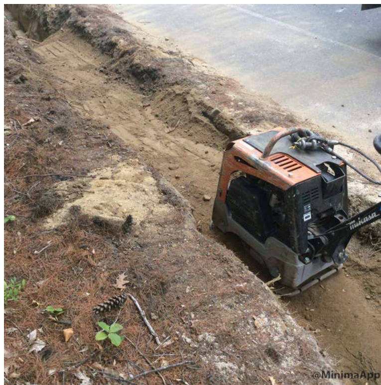
Compacting backfill with plate wacker
