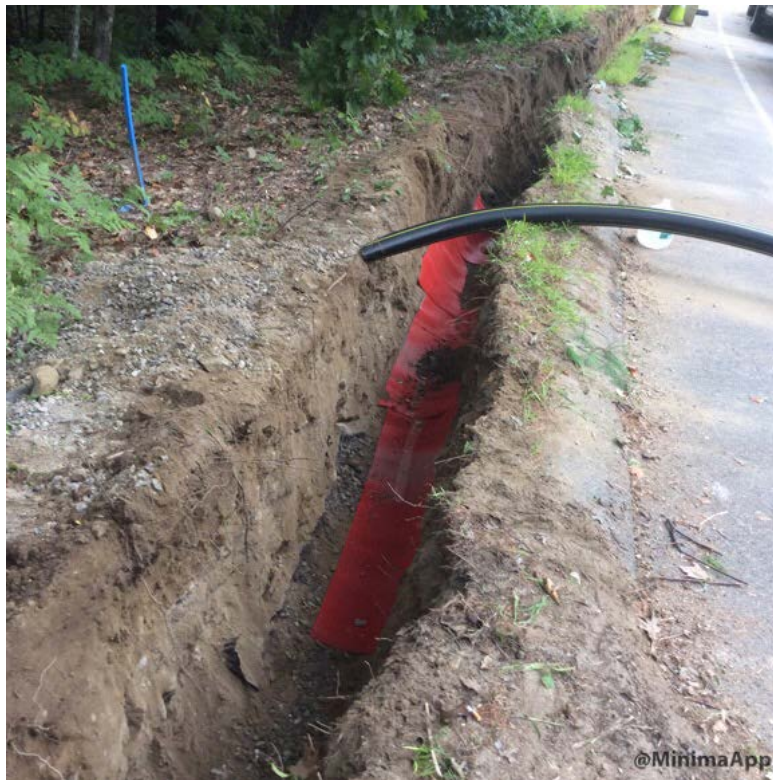
Rock shield place at the Stormdrain crossing
