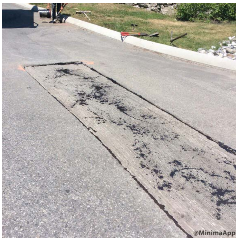
Milled area cleaned and tacked on Casco Bay Drive
