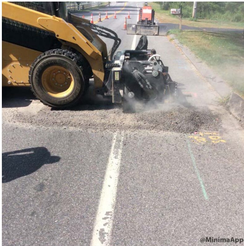
Milling trench patch on Route 88
