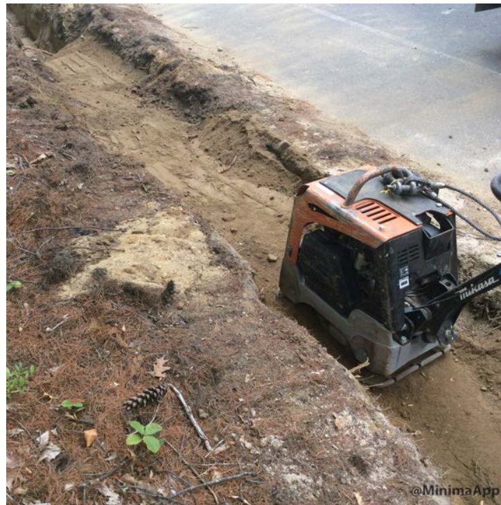
Compacting backfill with plate wacker
