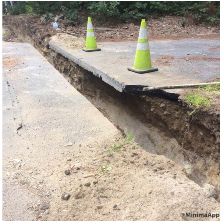
Driveway trench undermined at house #38
