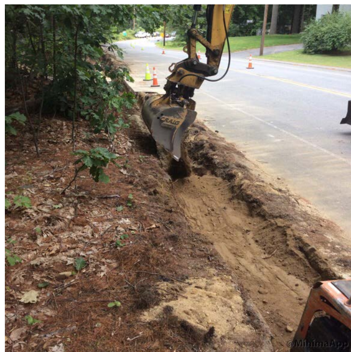
Placing backfill in trench
