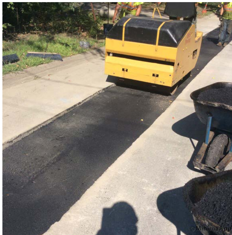
Compacting second lift of 12.5mm HMA with roller.
