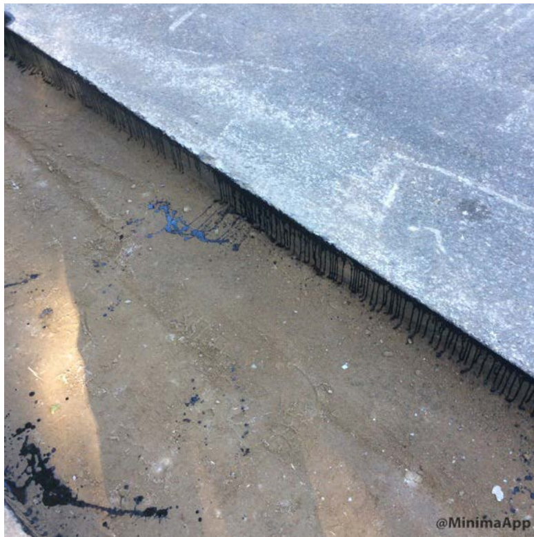
Tack placed on edge of existing pavement.
