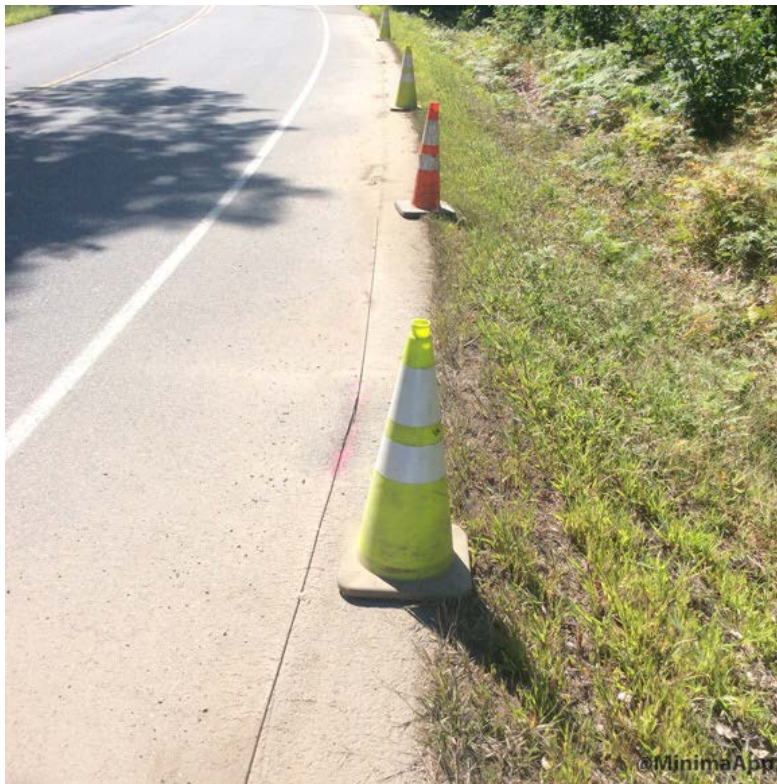
Sawcut pavement near large culvert
