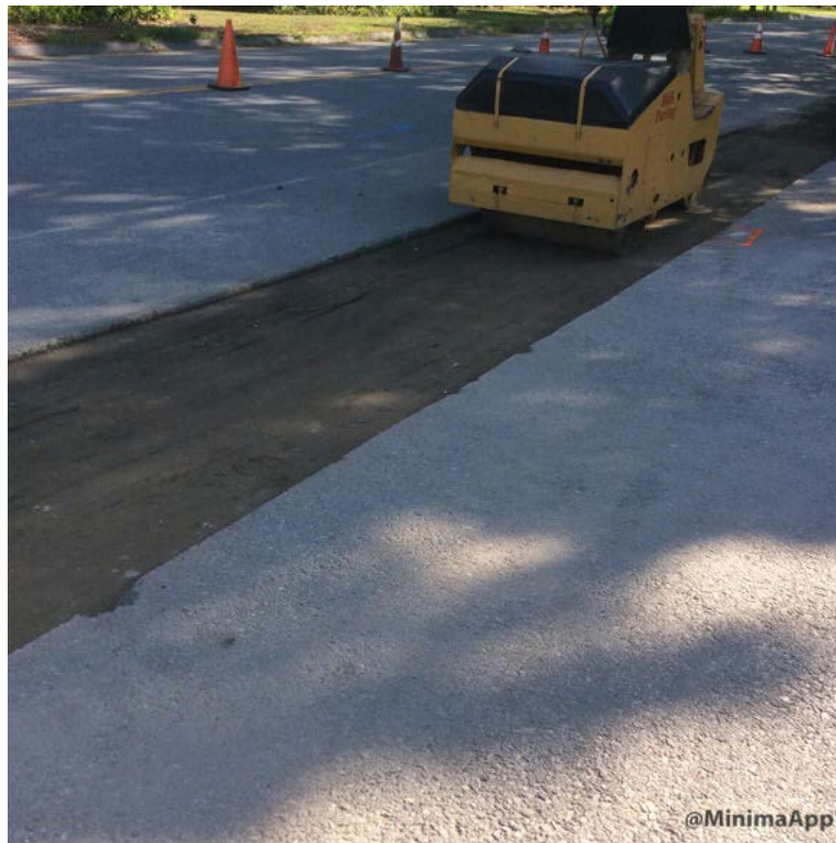
Compacting gravel with 3 ton vibratory roller.
