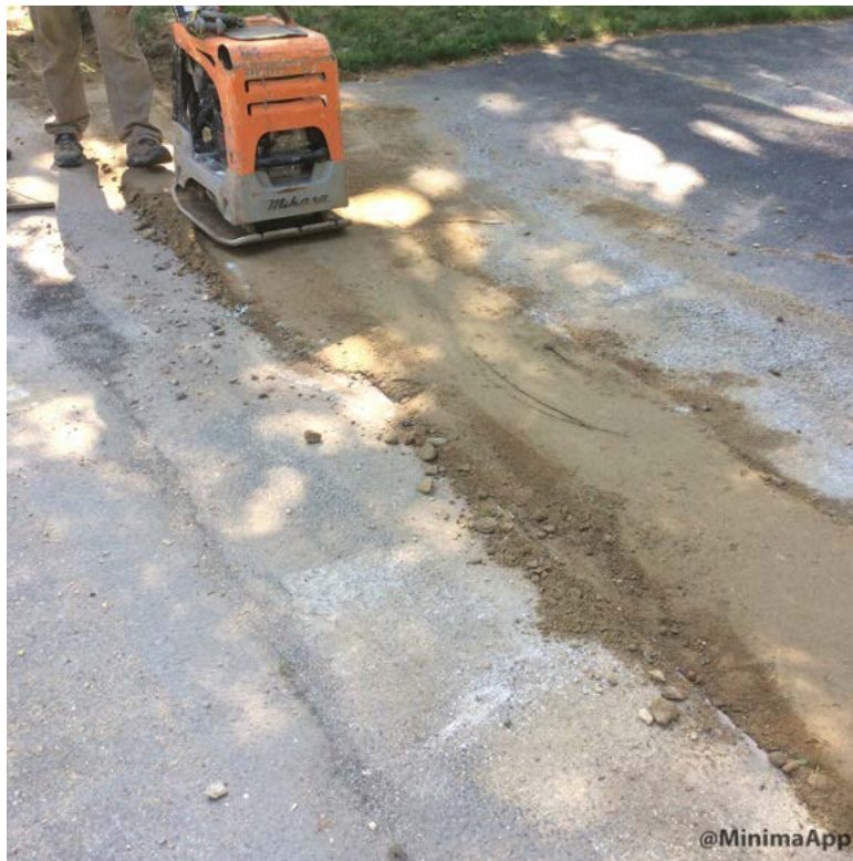
Compacting backfill at driveway crossing
