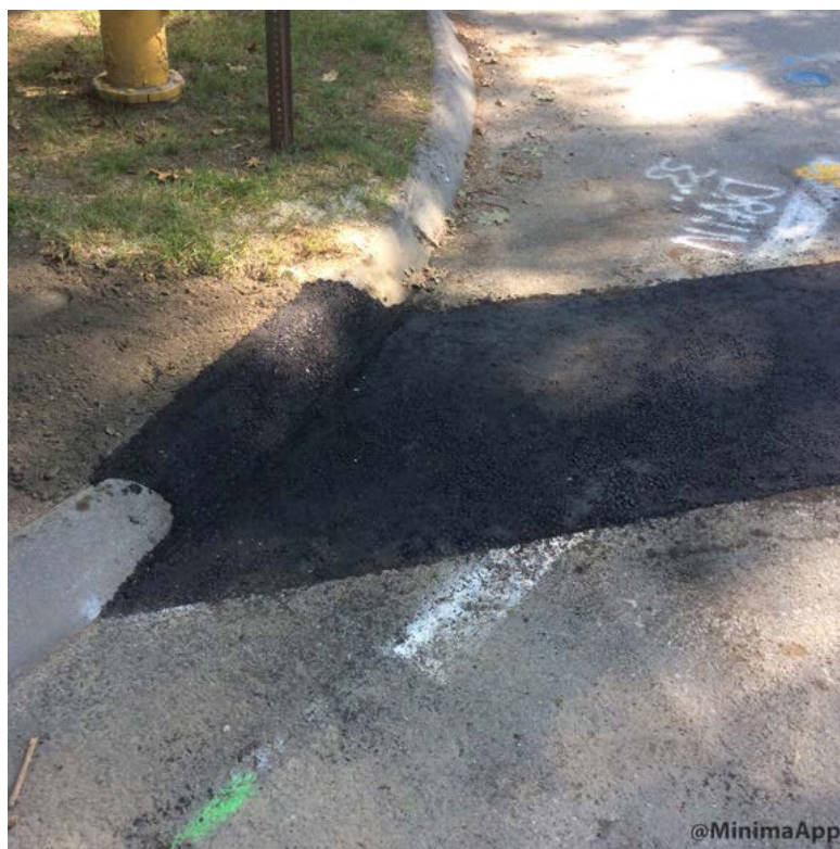
Hand built curb and completed trench at Kathy Lane.
