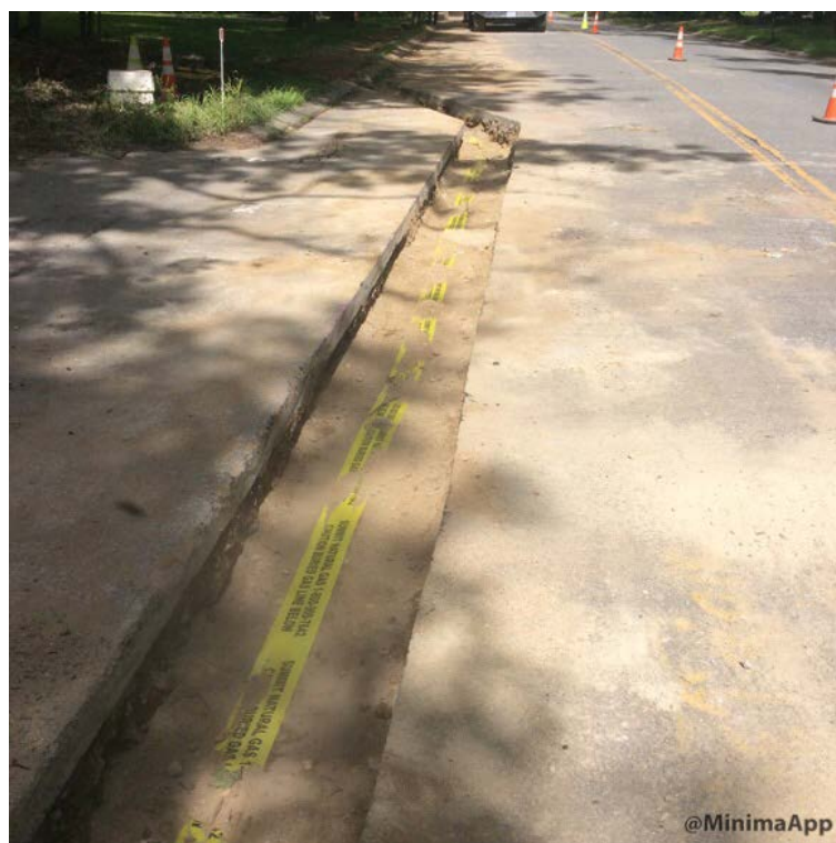
Roadway trench with second lift of backfill and warning tape.
