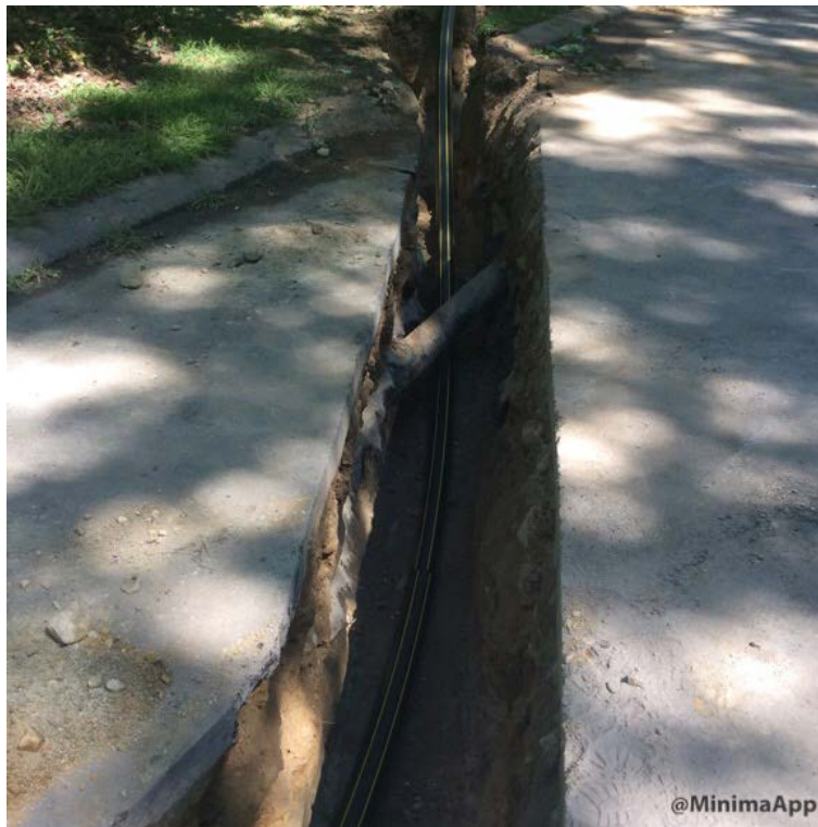
Gas main crossing under 6" underdrain.
