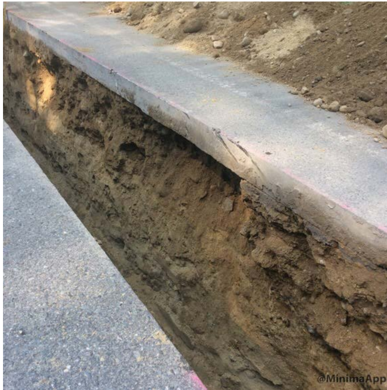
Area of some undermining along trench wall.
