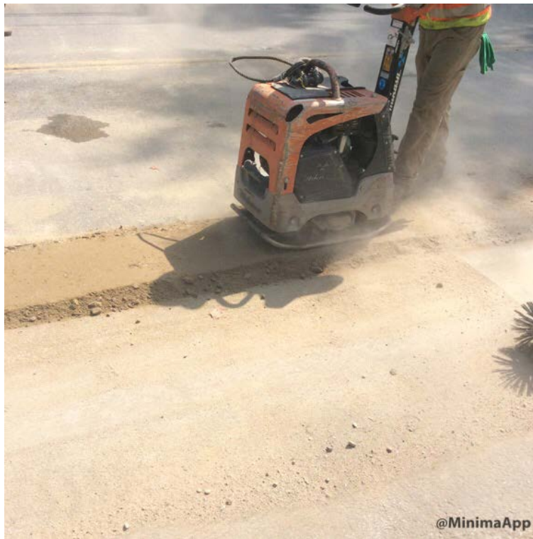
Compacting backfill with plate wacker.
