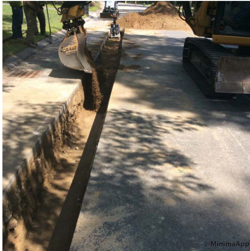
Backfilling roadway trench in the westbound lane on Skillin Road
