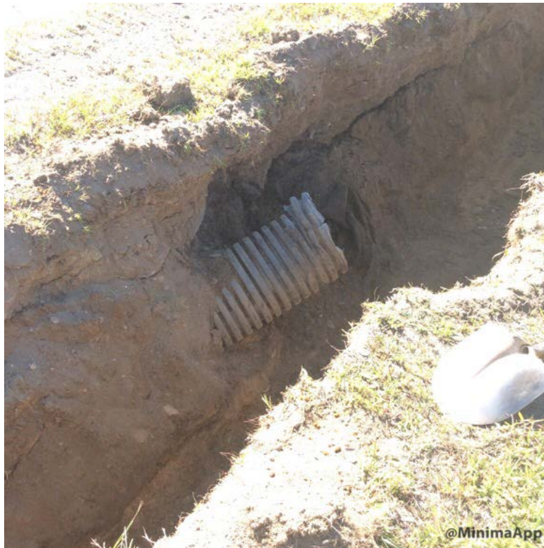
Damaged abandoned storm drain
