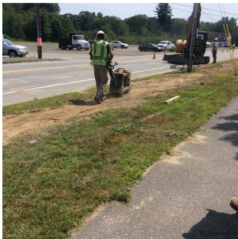
Compacting backfill with plate wacker
