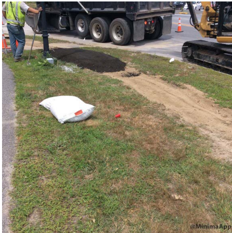
Placing loam in esplanade
