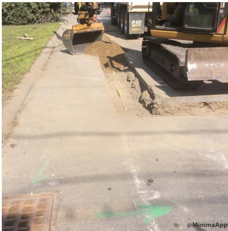
Crew placing backfill in roadway trench
