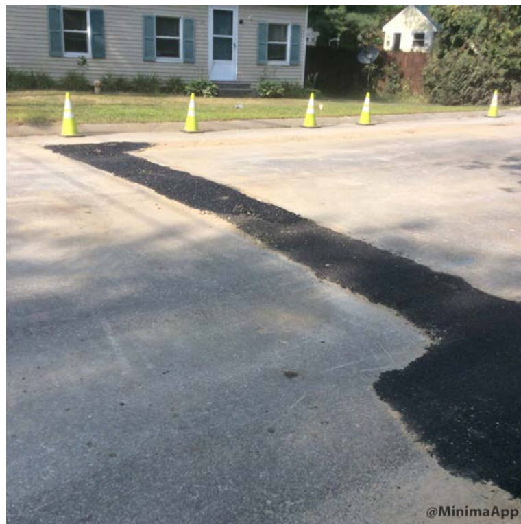
Cold patch in roadway crossing trench
