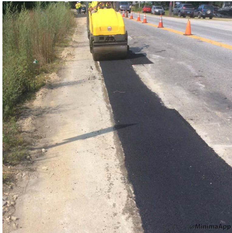
Compacting 12.5mm HMA with 3 ton roller
