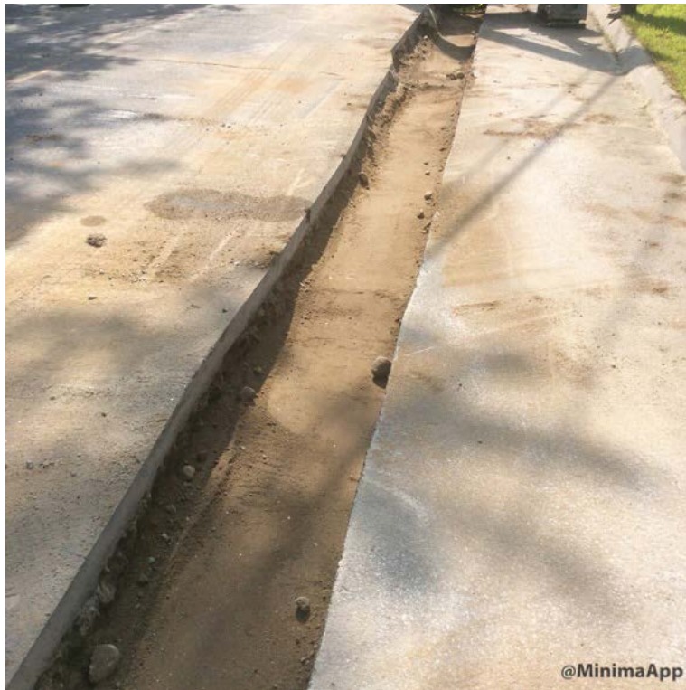
Backfill compacted in gas main trench
