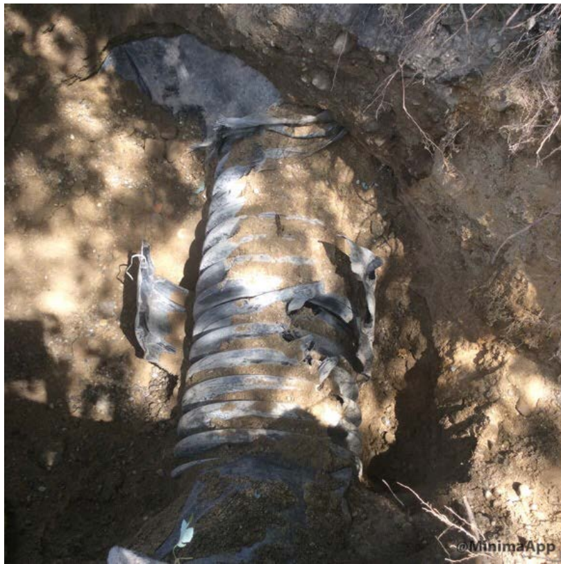
Damaged 24" stormdrain.
