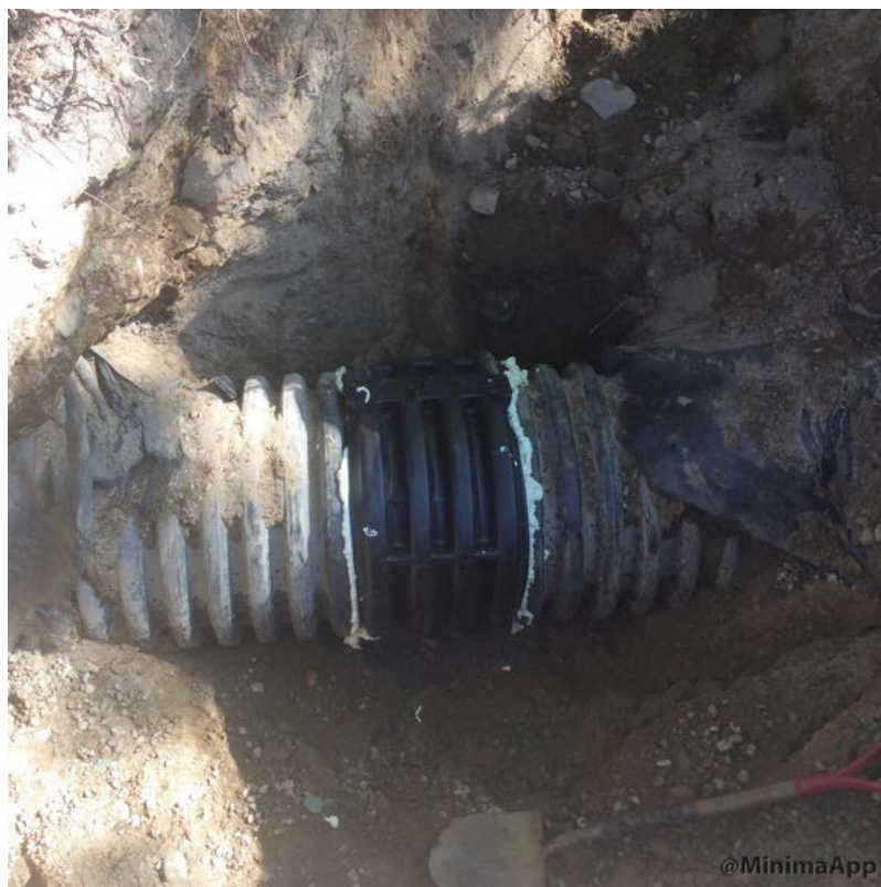
Stormdrain repaired with collar
