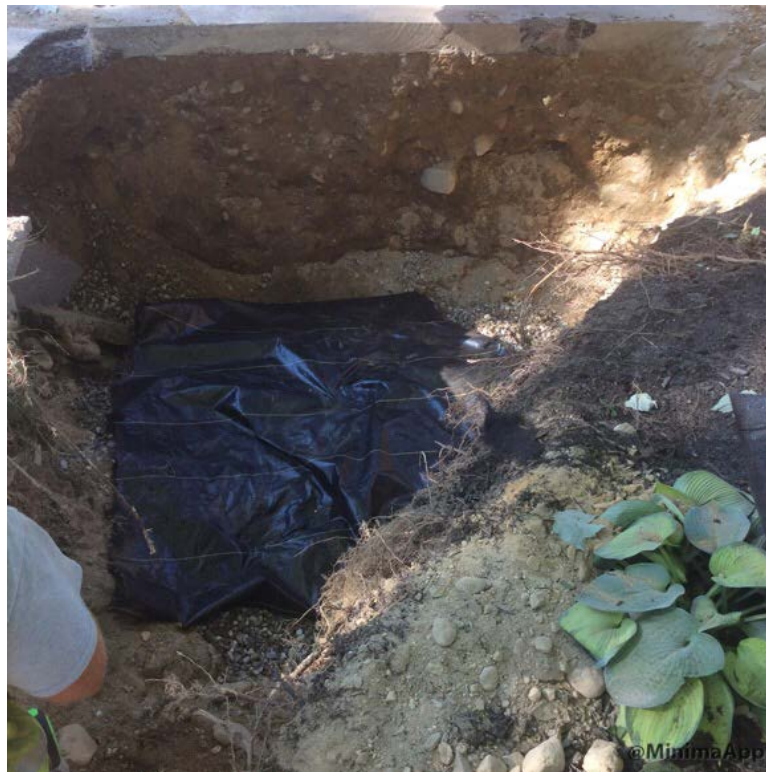
Fabric placed over crushed stone
