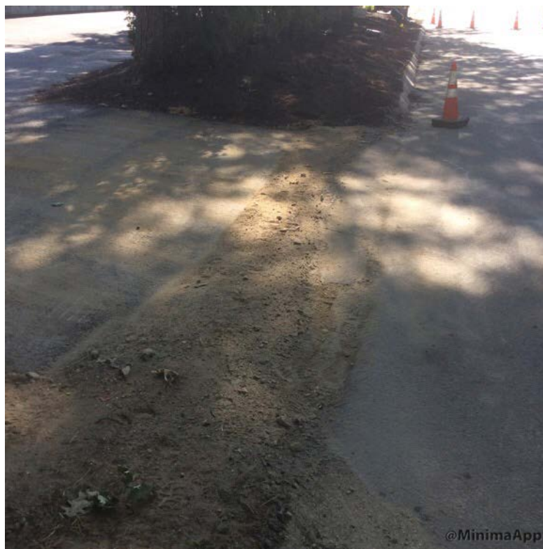
Backfill compacted at #5 driveway crossing
