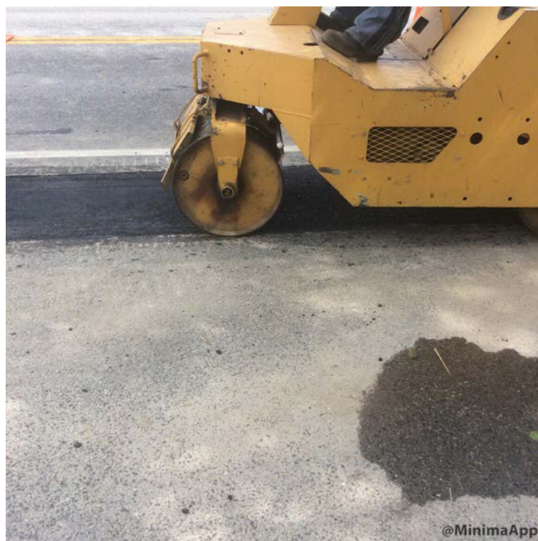
Compacting driveway crossing trench at Seymour's Bird Refuge
