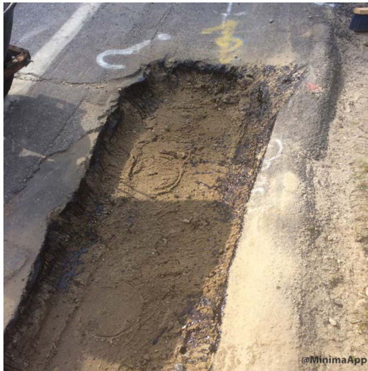
Gravel compacted and tack applied to edges of existing pavement.
