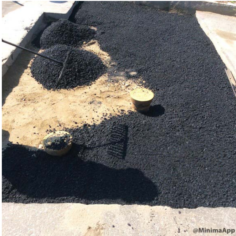
Placing 12.5mm HMA in trench at the corner of Blackstrap Road
