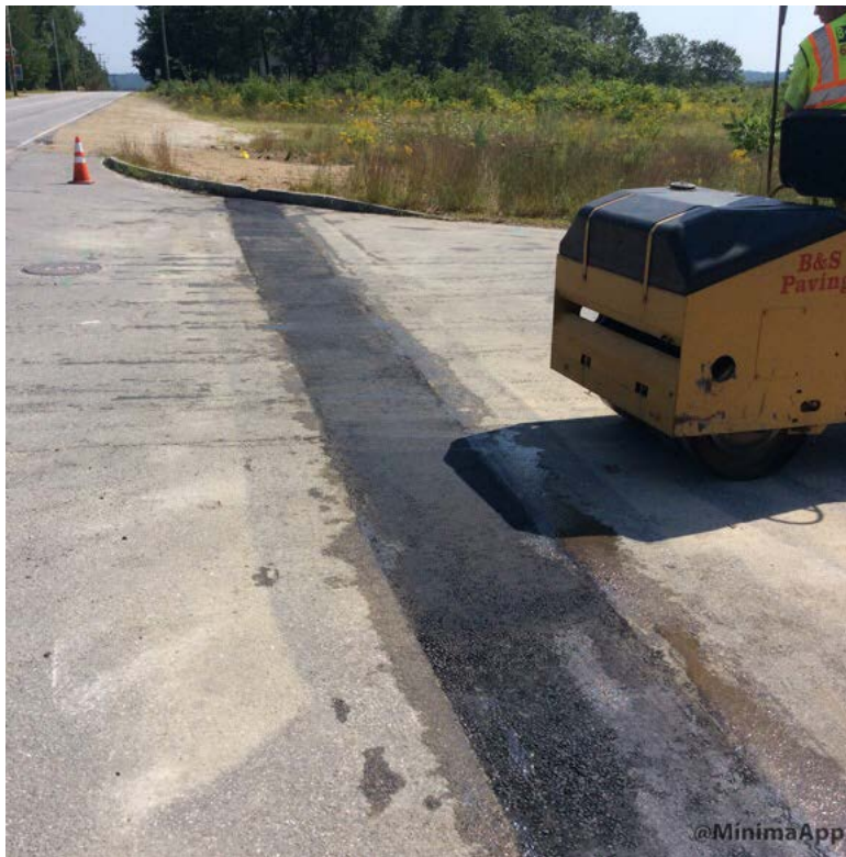
Compacting 12.5mm HMA with 3 ton roller at Westside Animal Hospital
