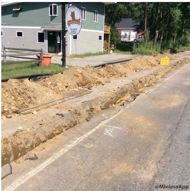
Longitudinal roadway trench for gas main install
