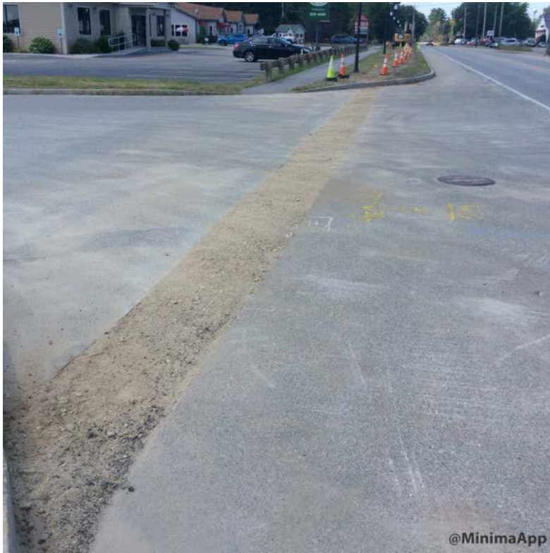
Gravel pit driveway trench backfilled with gravel
