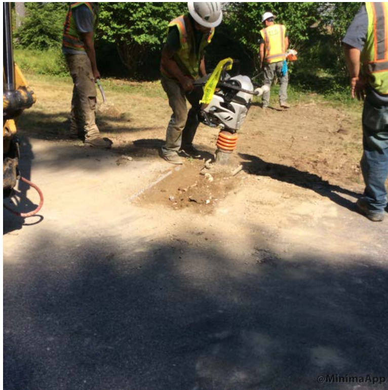
Compacting gravel on Friar Lane
