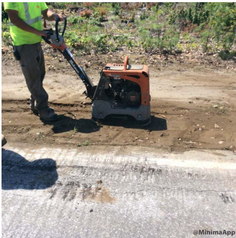
Compacting backfill on Route 100
