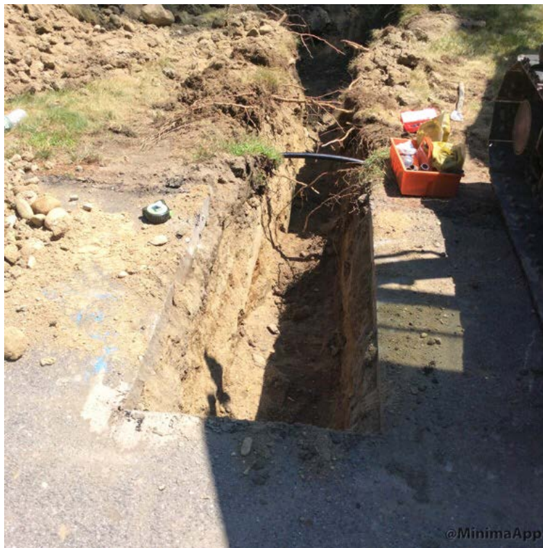
Roadway trench on Friar Lane for Water Main location
