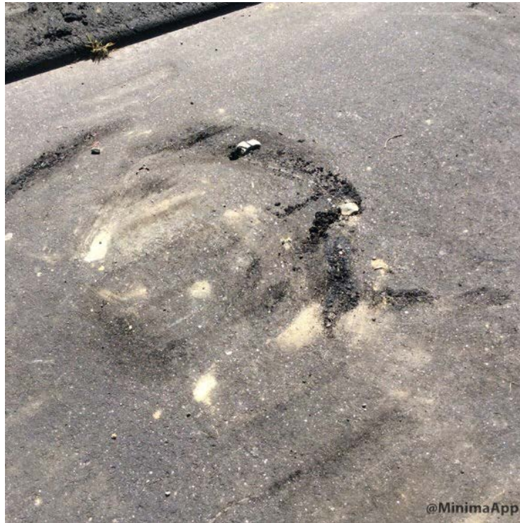
Roadway damaged by excavator tracks
