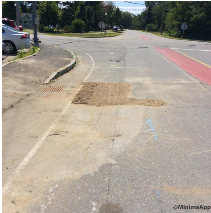
Trench backfilled on Skillin Road
