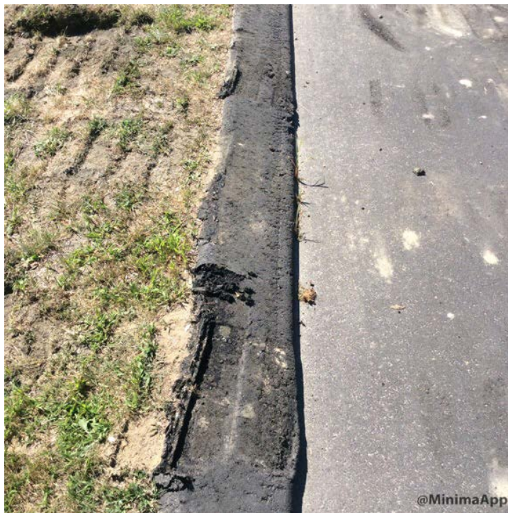
Curb damaged by excavator tracks
