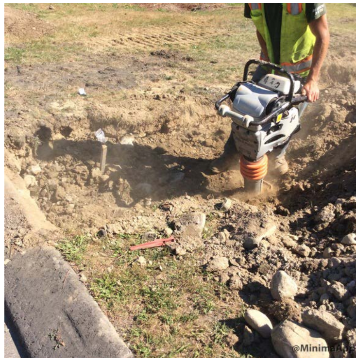
Compacting backfill with jumping jack
