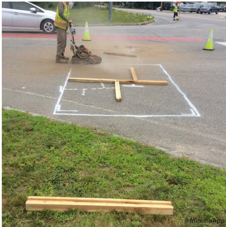
Crew saw-cutting area on on Blackstrap Road
