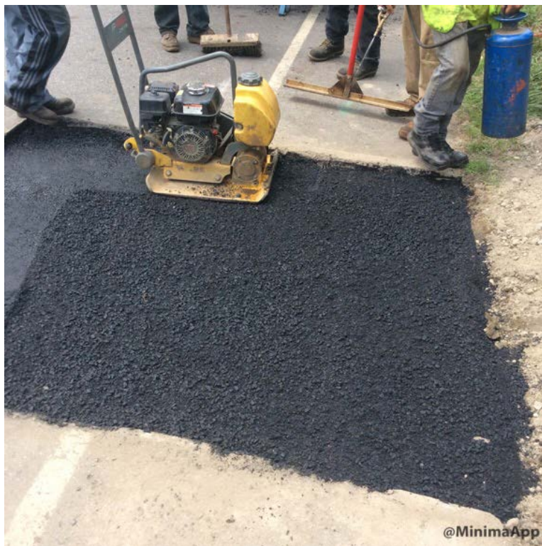
Compacting first lift of 12.5mm HMA
