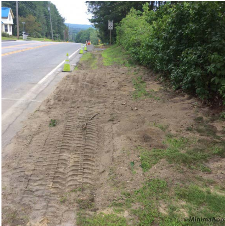
Drill machine trench backfilled
