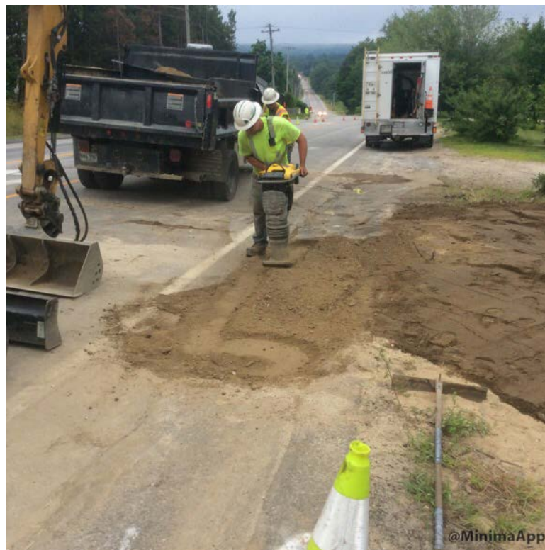
Compacting final lift of backfill with jumping jack
