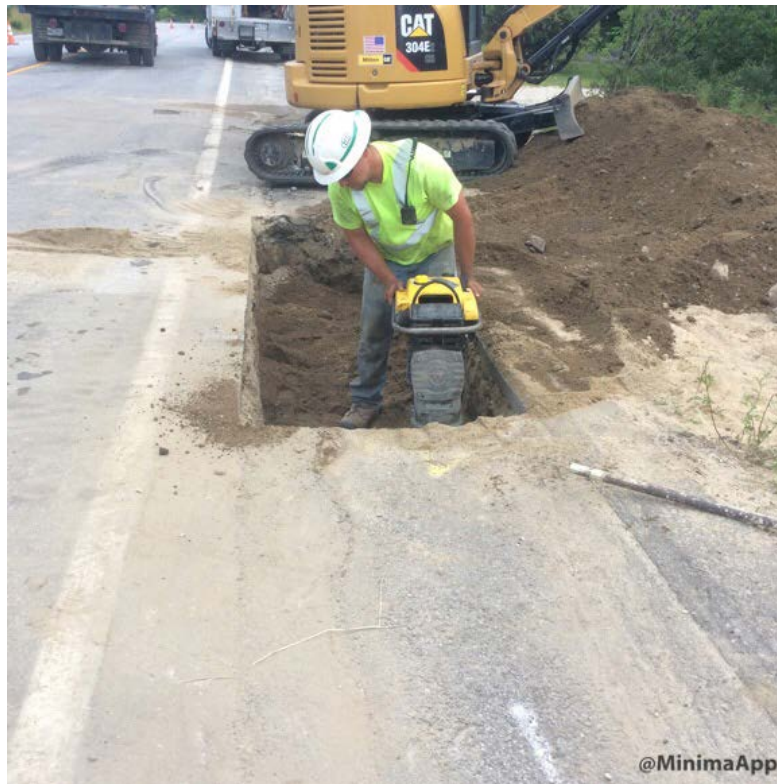
Compacting backfill with jumping jack.
