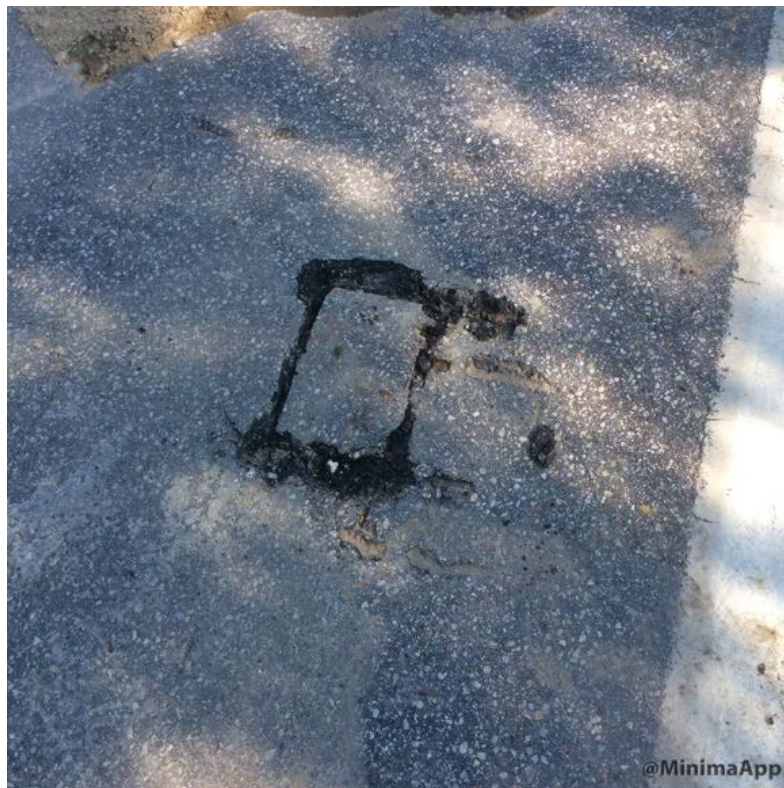
Damaged pavement in travel way from drill machine near CMP pole 3.I.
