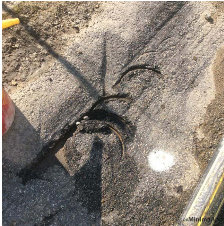
Damaged pavement in paved swale area from drill machine near CMP pole 3.I.
