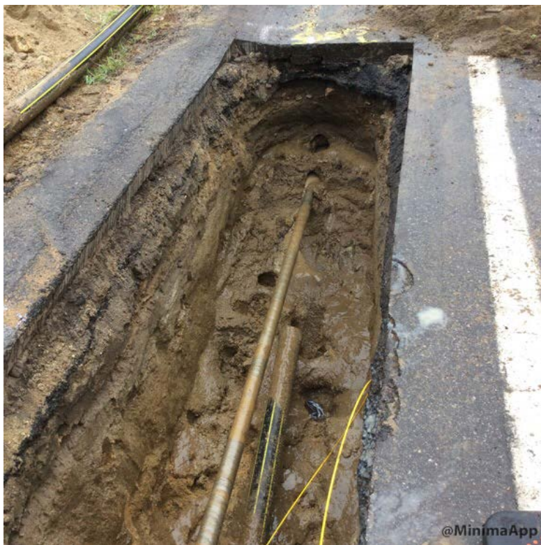
Shoulder trench for direction drill machine
