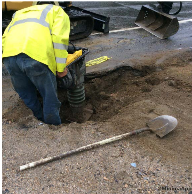
Compacting backfill with jumping jack
