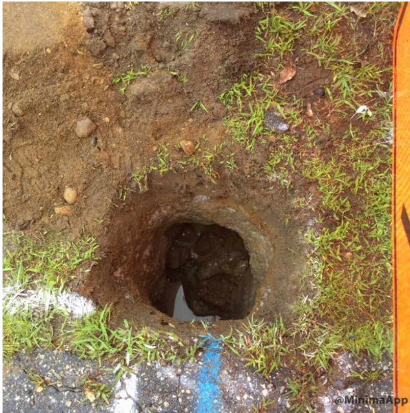
Pot hole to locate water service
