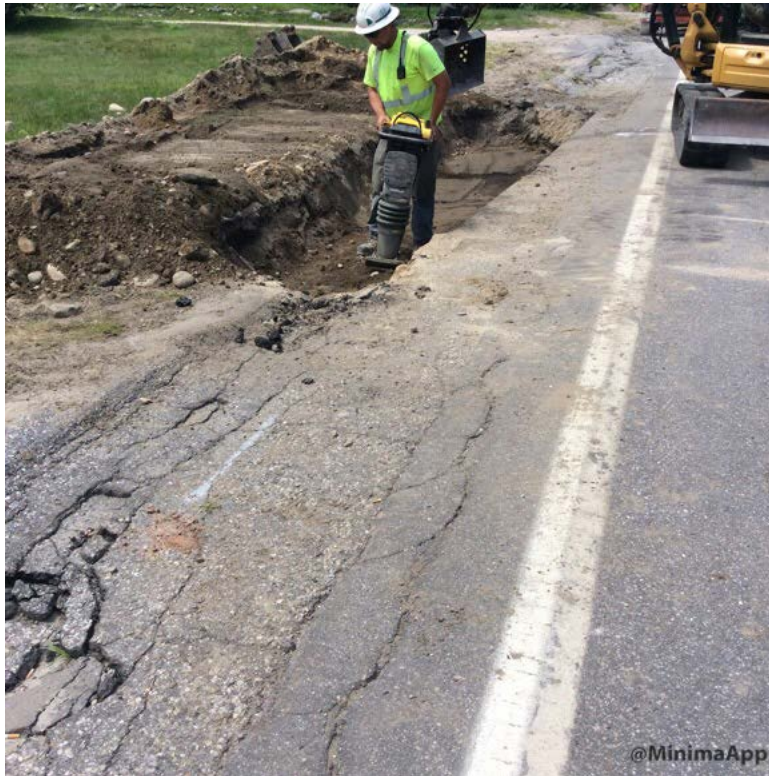
Compacting second lift of gravel near lower driveway to house #144
