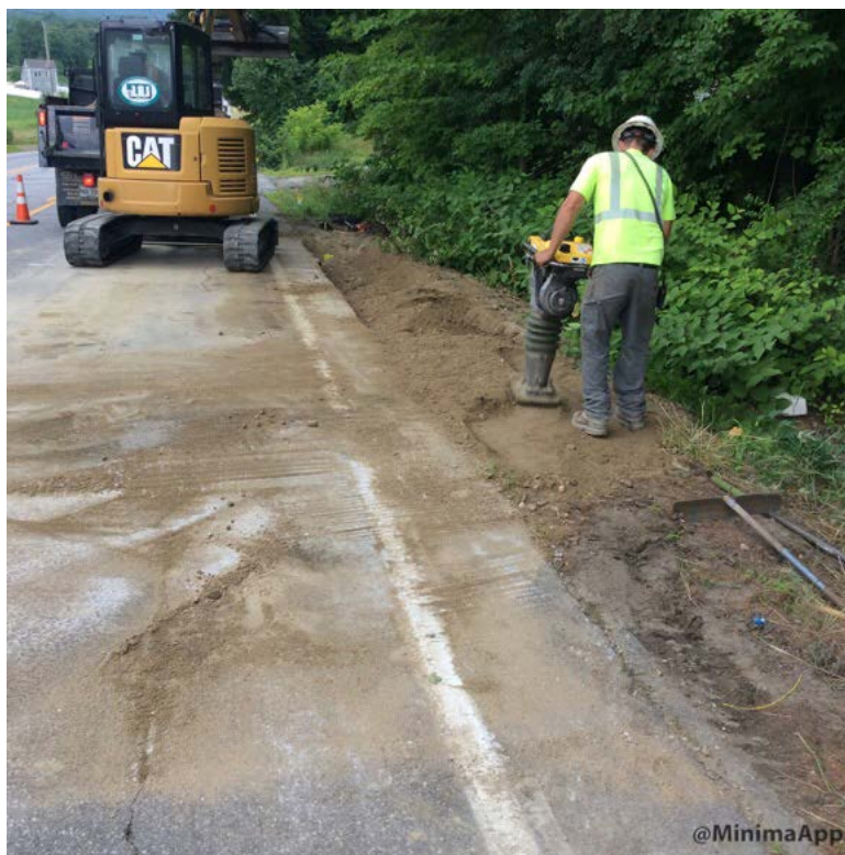
Compacting final lift of gravel near house #134
