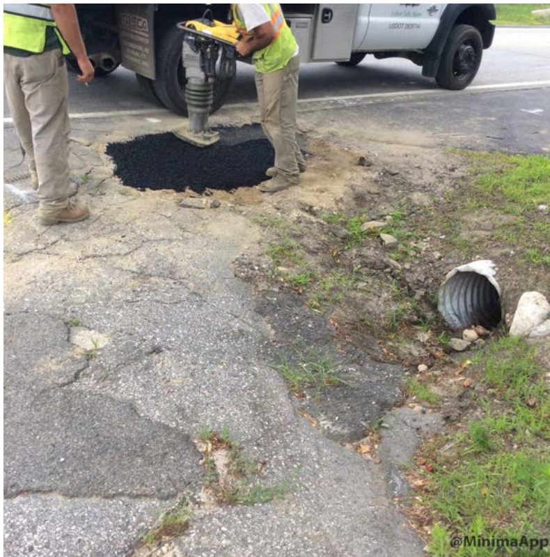
Compacting cold patch at corner of Spring Drive
