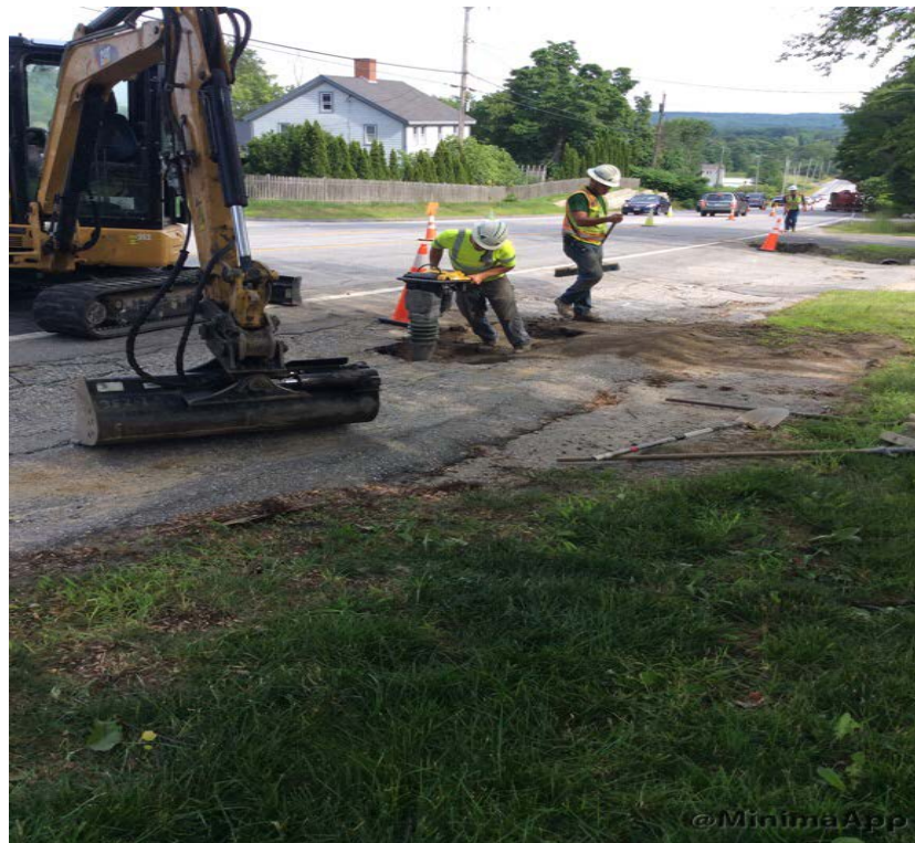
Compacting road near #138 water service on Rt. 100
