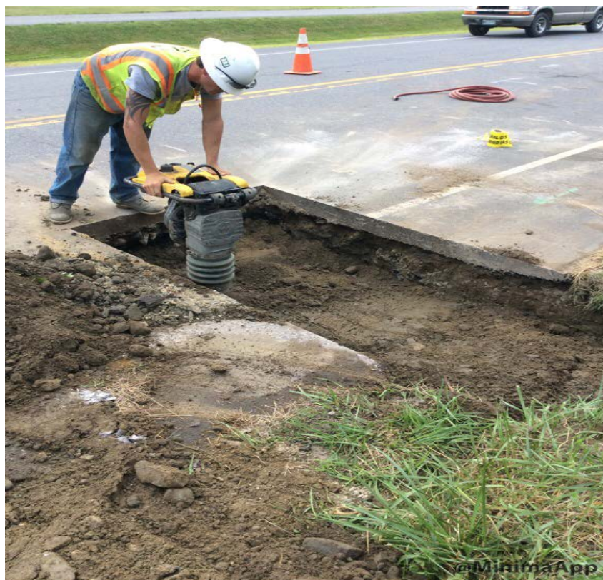
Compacting backfill on Tuttle road
