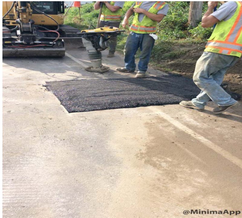
Cold patch placed at Tuttle Road
