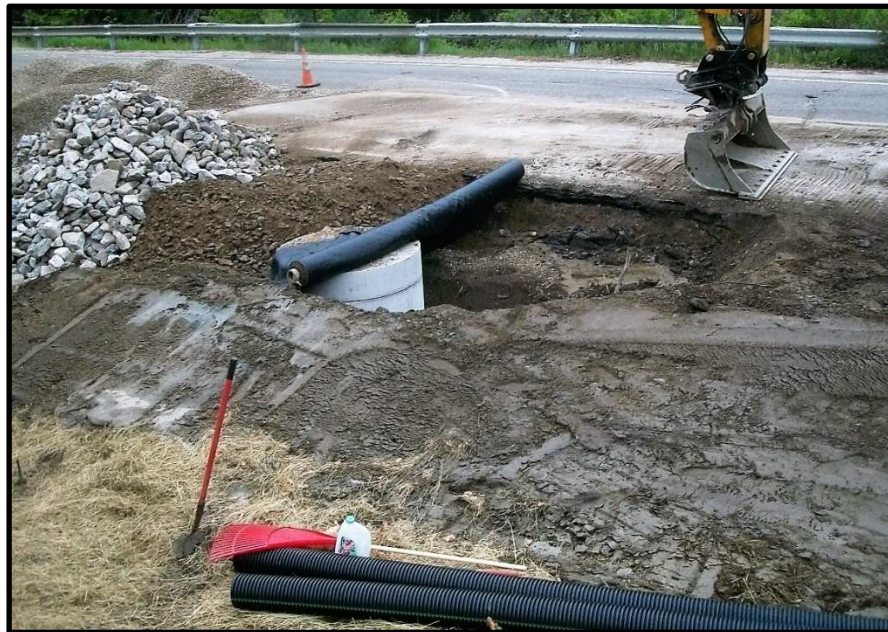
Photograph 8: Catch basin CB-5G at STA 57+15 and rip rap outlet prior to the installation of 6-inch underdrain (foreground) from the inlet uphill (northward).
