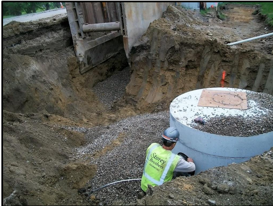
Photograph 2: At the end of the day placed filter fabric over openings in CB-6B prior to placing backfill at STA 63+50.
