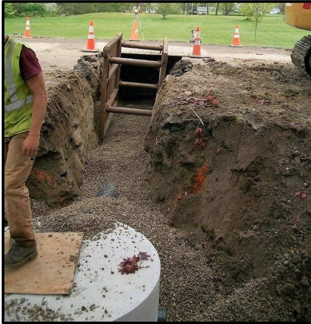
Photograph 5: 12-inch storm drain crossing road between CB-6E (foreground in front of Maloney lot) and CB-6B (far side of road in front of Soule lot).
