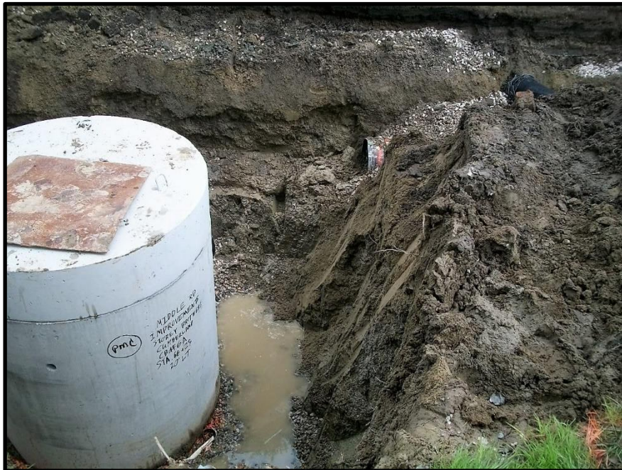
Photograph 4: Catch Basin CB-6A installed per plan prior to connection of 12-inch underdrain outlet.
