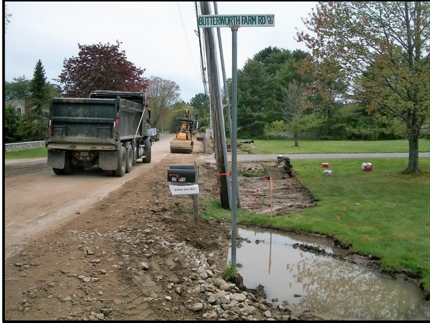
Photograph 3: Compacted Type D gravel placed over crushed stone to grade behind underdrain installation.
