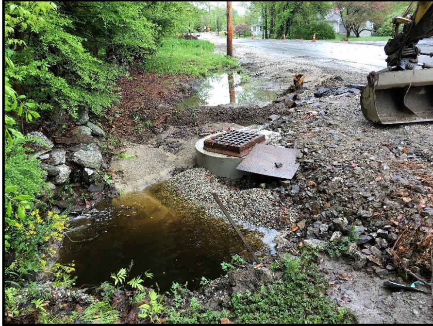
Photograph 9: Due to ponding after heavy overnight rains May 25-26 th a grate was placed over the opening of the structure for CB-7E at STA 78-28 to improve surface drainage.
