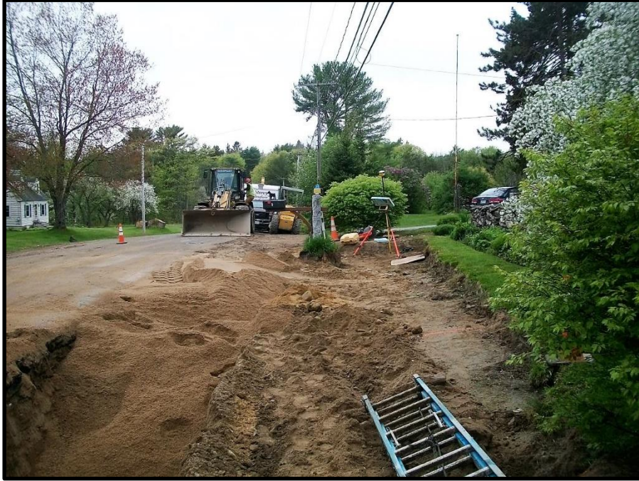
Photograph 1: Installed 15-inch underdrain and placed sand backfill over fabric at 122 Middle.
