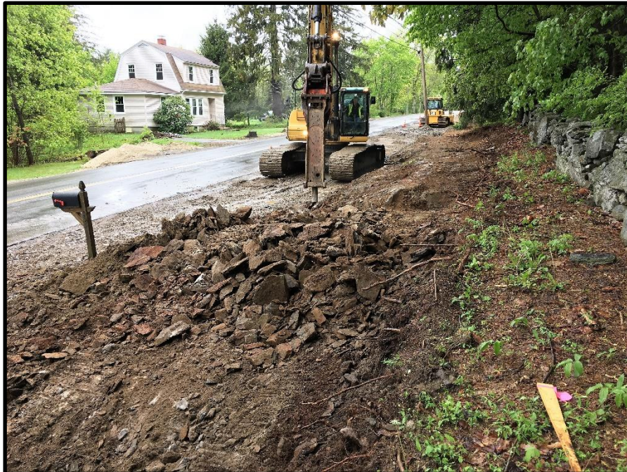
Photograph 10: Work Friday, May 26 th was largely limited to ledge removal across the road from 147 & 151 Middle Road.
