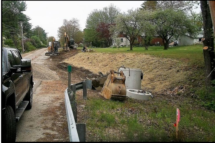
Photograph 7: Stump removal and geotextile reinforced slope at 117 Middle Road (Casey) prior to installation of catch basin CB-5G.
