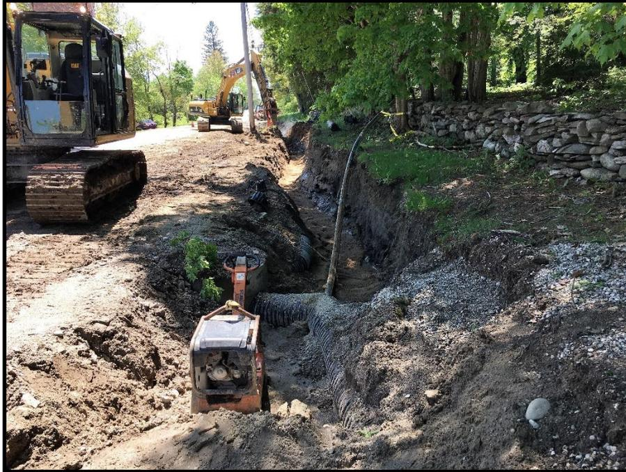
Photograph 5: Routing gas line behind CB-8B. Ledge removal in background.
