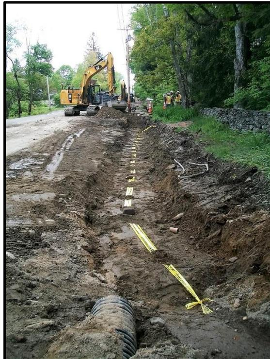
Photograph 8: Warning tape 24 inches above gas line south of existing 12-inch underdrain inlet at STA 80+15 looking southward.
