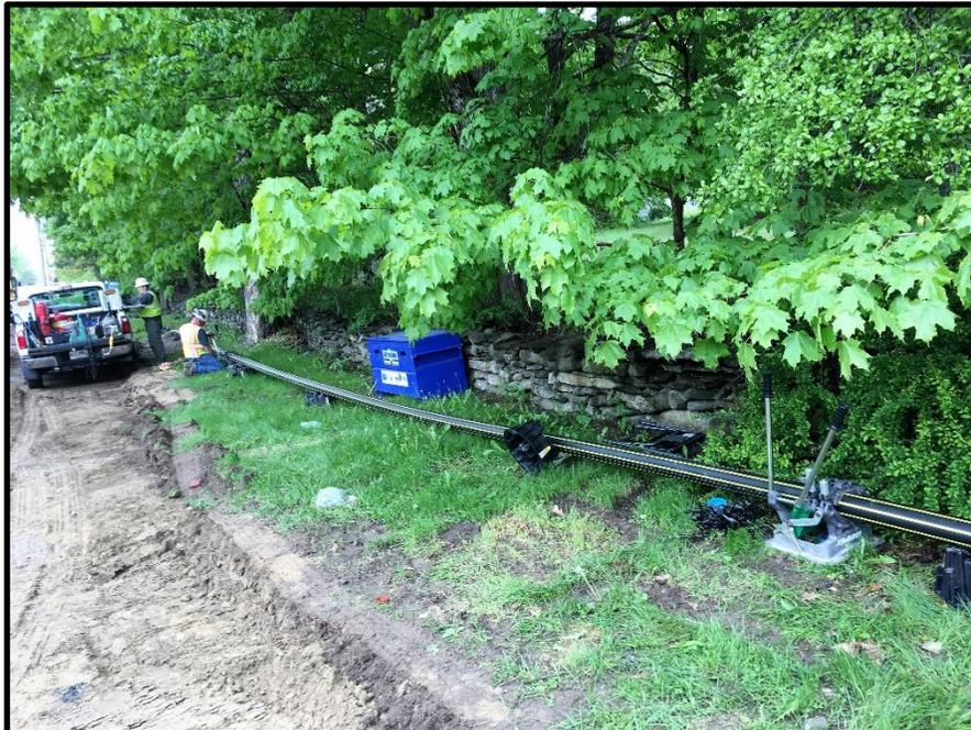
Photograph 2: Sections of pipe being fused together and staged for installation.
