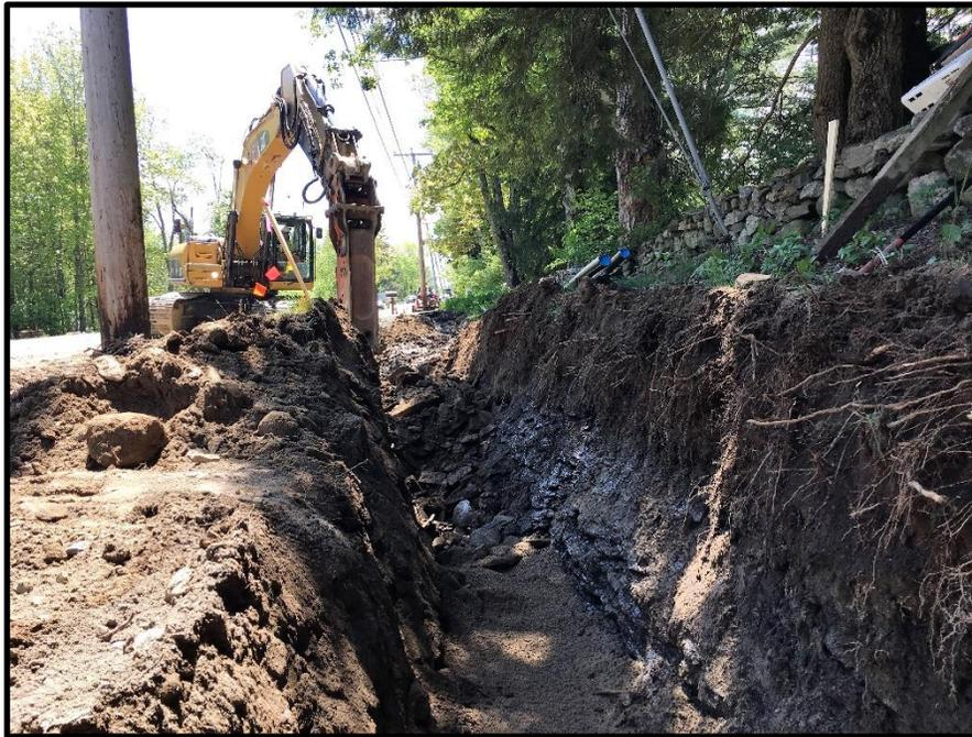
Photograph 6: Ledge removal behind Pole #339 at STA 80+30.
