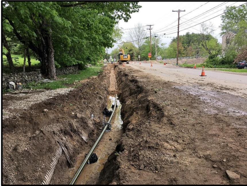
Photograph 3: First segment of pipe placed from Tuttle Road. Existing 12-inch underdrain in foreground.
