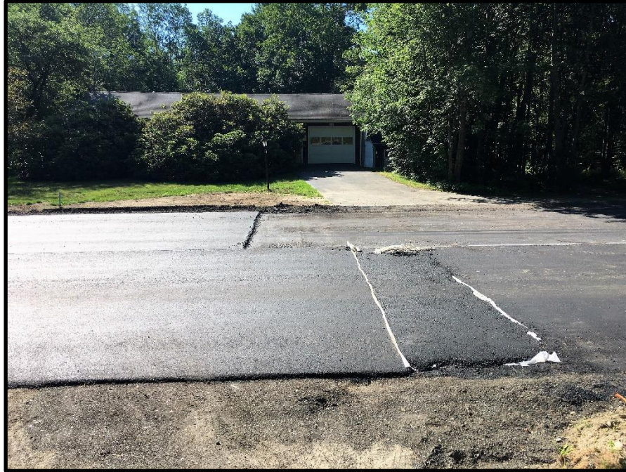
Photograph 11: When paving resumed Wednesday, July 5 th the temporary pavement ramp was removed on the northbound lane being paved in the morning at STA 79+00 but remained in southbound lane until paving switches to southbound lane in the afternoon.
