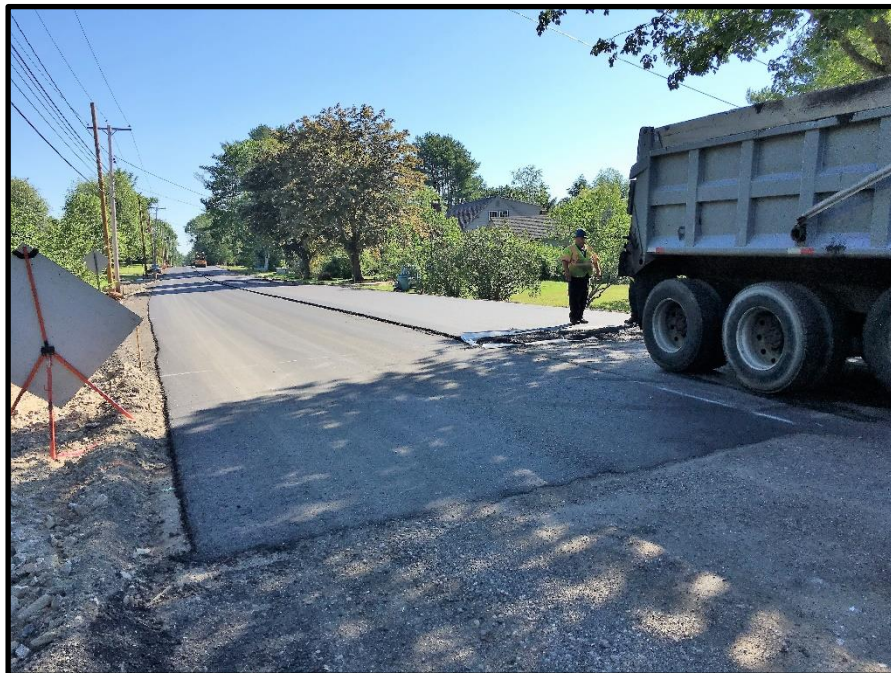
Photograph 12: After completing the 2 nd layer of pavement in the northbound lane, a temporary paved ramp was installed at STA 62+00 prior to opening the lane to traffic and switching over to pave the southbound lane. A second temporary ramp was installed later in the southbound lane.
