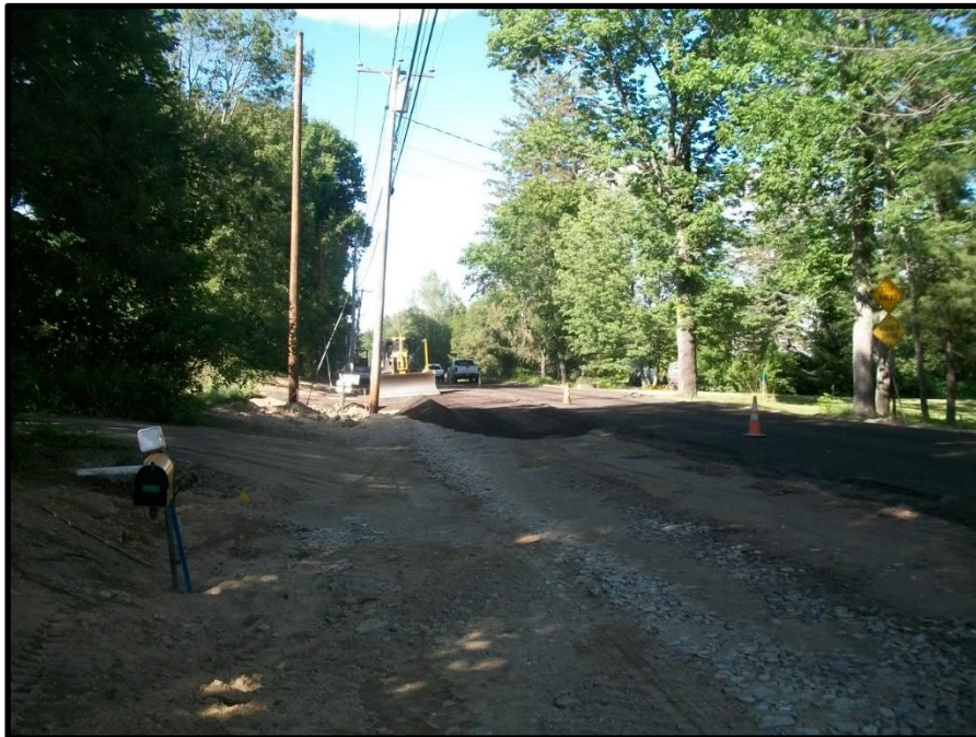
Photograph 2: Placed reclaimed pavement millings in the afternoon of Monday, 6/26 from 146 Middle Road to 137 Middle Road.
