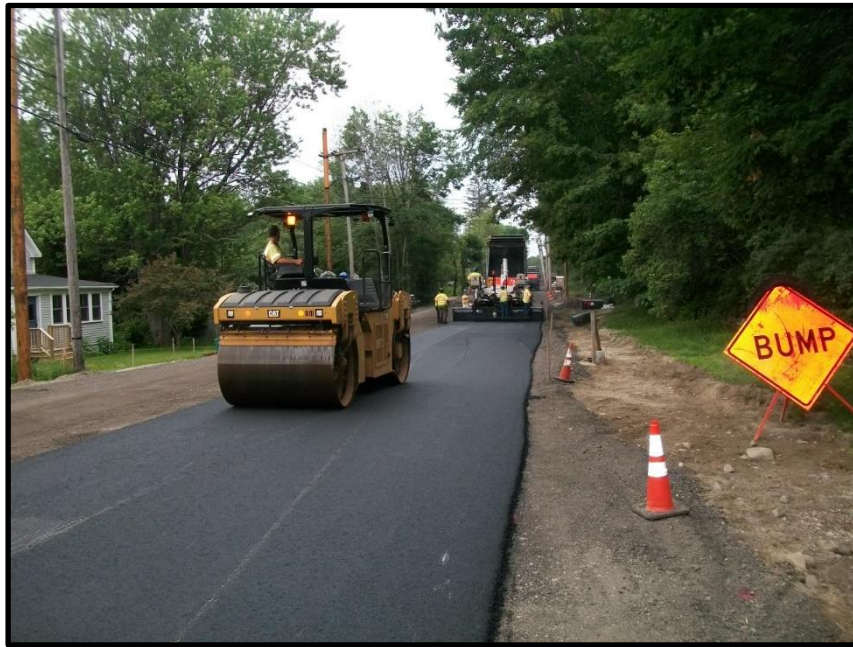
Photograph 7: Knockdown roller following behind the paver soon after paving operations got underway on the morning of Thursday, June 29 th .
