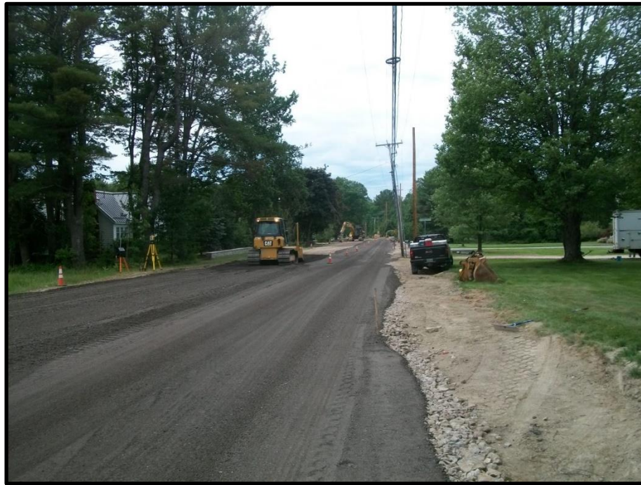
Photograph 3: Placing millings on east side of road in a southerly direction near Butterworth Farm Road on the morning of Tuesday, June 27 th .
