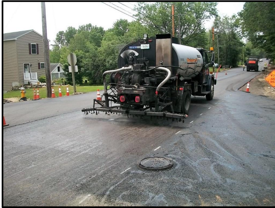
Photograph 9: Tack truck spraying the pavement surface prior to placing the 2nd layer of pavement on Friday, June 30 th . Paving was limited to the afternoon only due to morning rains.
