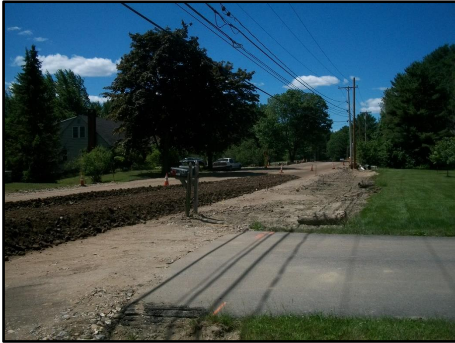
Photograph 1: Placed additional Type D gravel on the morning Monday, June 26 th from 140 Middle Road to 126 Middle Road.
