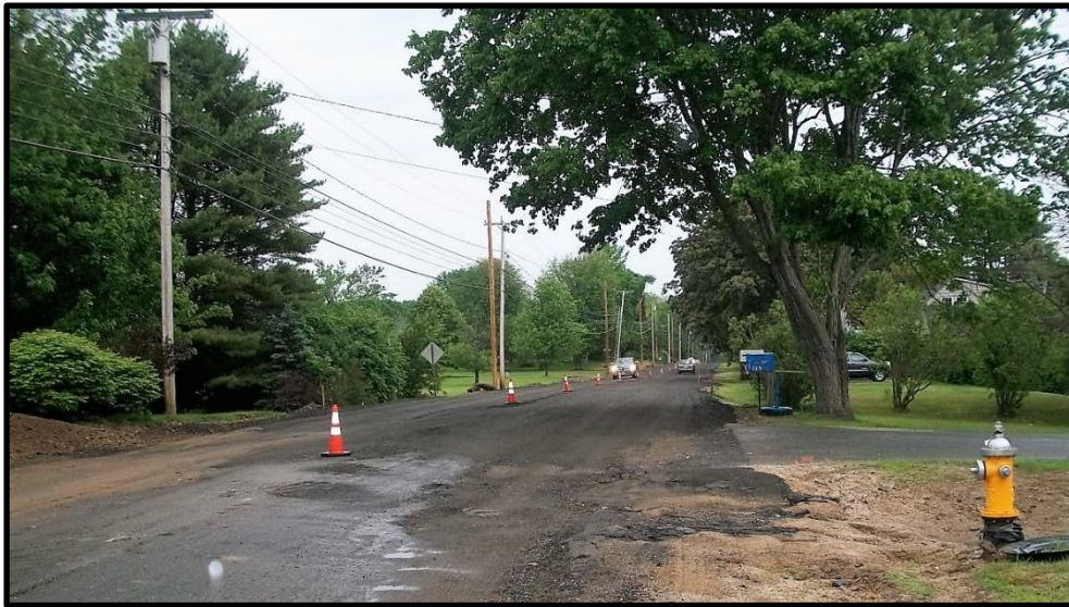
Photograph 4: Finished placing pavement millings at the southern terminus to be paved at STA 61+75 (Casey driveway at 121 Middle Road) on Tuesday afternoon June 27 th .
