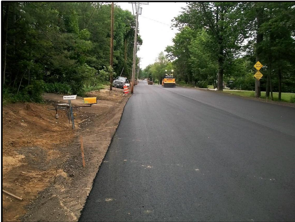
Photograph 8: View near the end of the day Thursday, June 29 th looking north depicting the rubber tire roller which follows behind the knockdown roller. Finishing roller in background.
