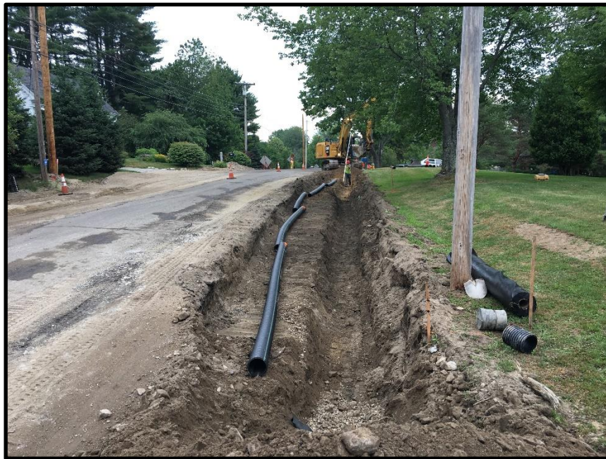
Photograph 4 – Tuesday, July 11 th : Completing the installation of 6-inch underdrain in east shoulder in front of Casey property.
