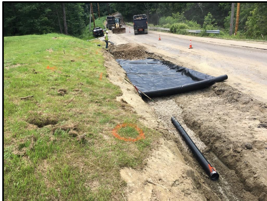
Photograph 2 – Monday, July 10th: Installing 6-inch underdrain in shoulder just north of Cherner Brook in front of Casey property.
