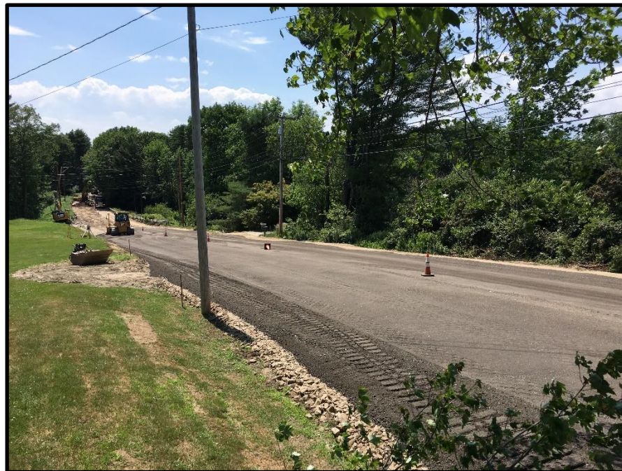
Photograph 6 – Wednesday, July 12 th : Stripping old pavement and re-establishing road base with Dozer and Roller.
