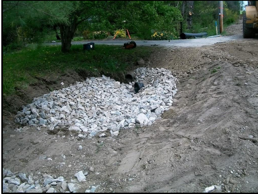
Photograph 9: Outlet of 15-inch underdrain south of driveway for 116 Middle Road near STA 58+65.
