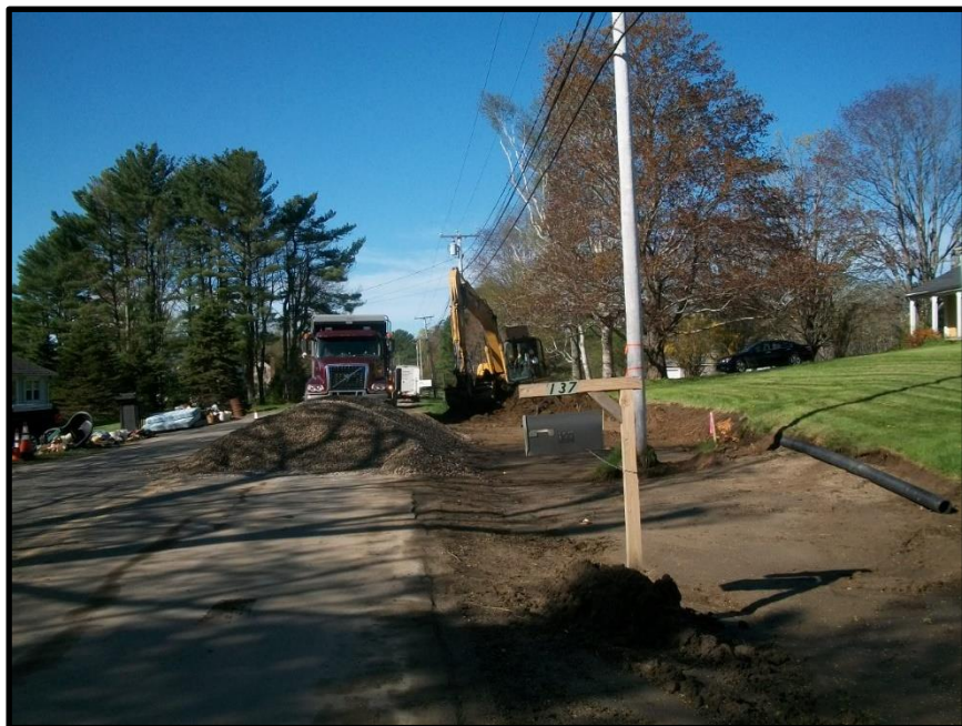
Photograph 3: Stripping and rough grading at Butterworth Farm ahead of underdrain installation.
