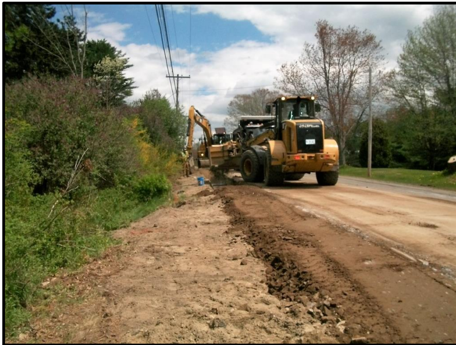
Photograph 10: Placing Type D gravel backfill over 15-inch underdrain south of 122 Middle Road.
