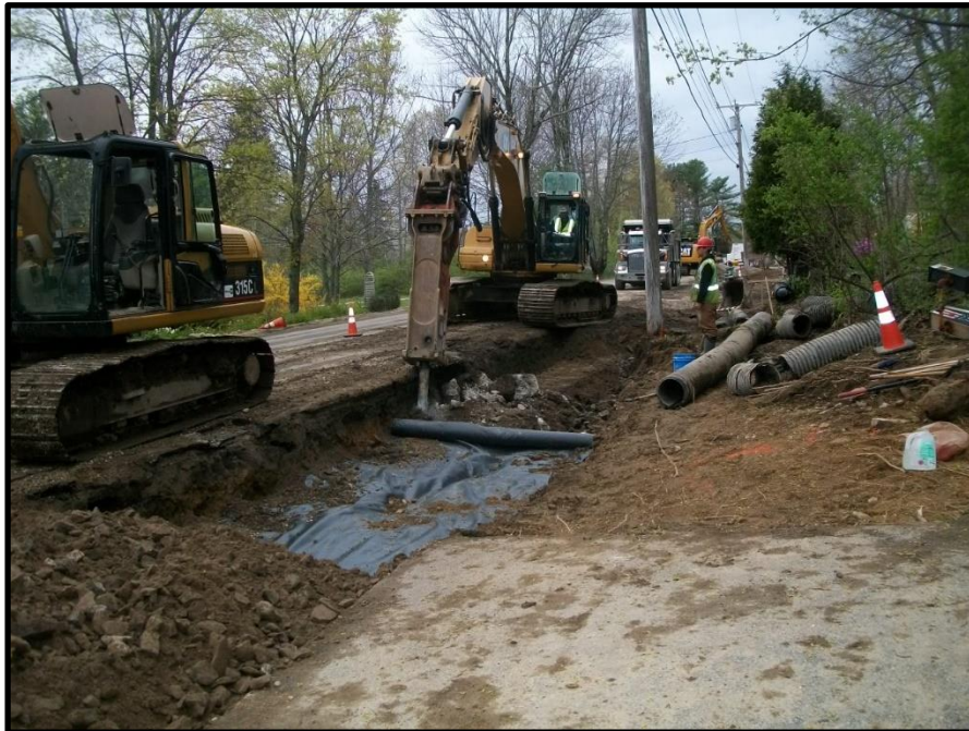
Photograph 2: Shallow ledge as high as road subgrade at STA 73+15 in front of 146 Middle Road.
