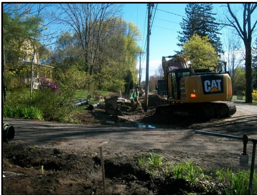
Photograph 4: Installation of 12-inch underdrain from 142 to 140 Middle Road.
