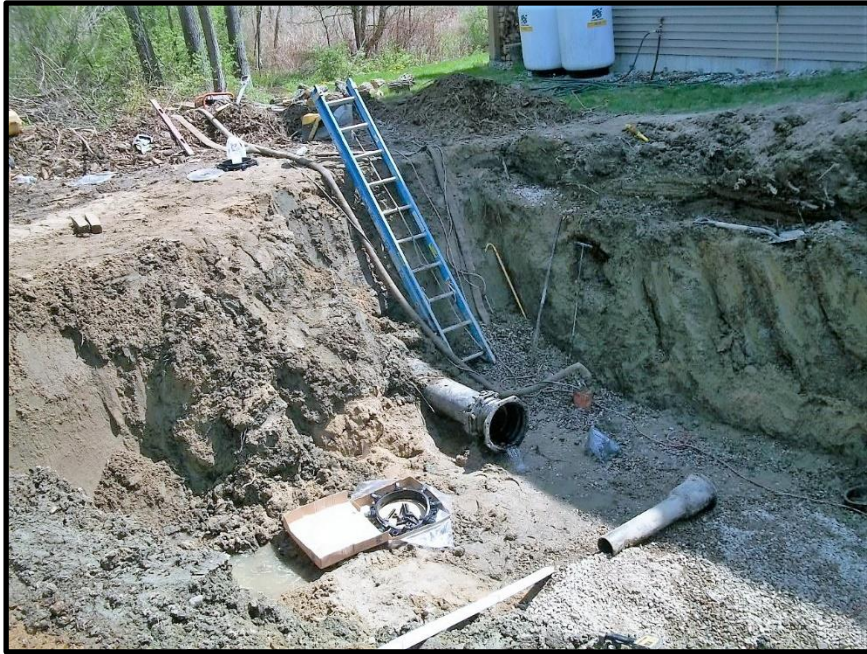
Photograph 5: 12"x10" adapter installed on existing 10-inch water main that runs parallel to Tuttle in side yard of 163 Middle Road.
