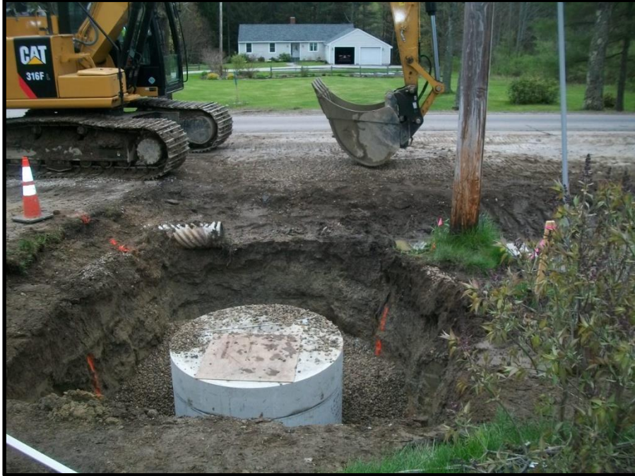
Photograph 1: Structure for catch basin CB-7B just south of 142 Middle Road driveway.
