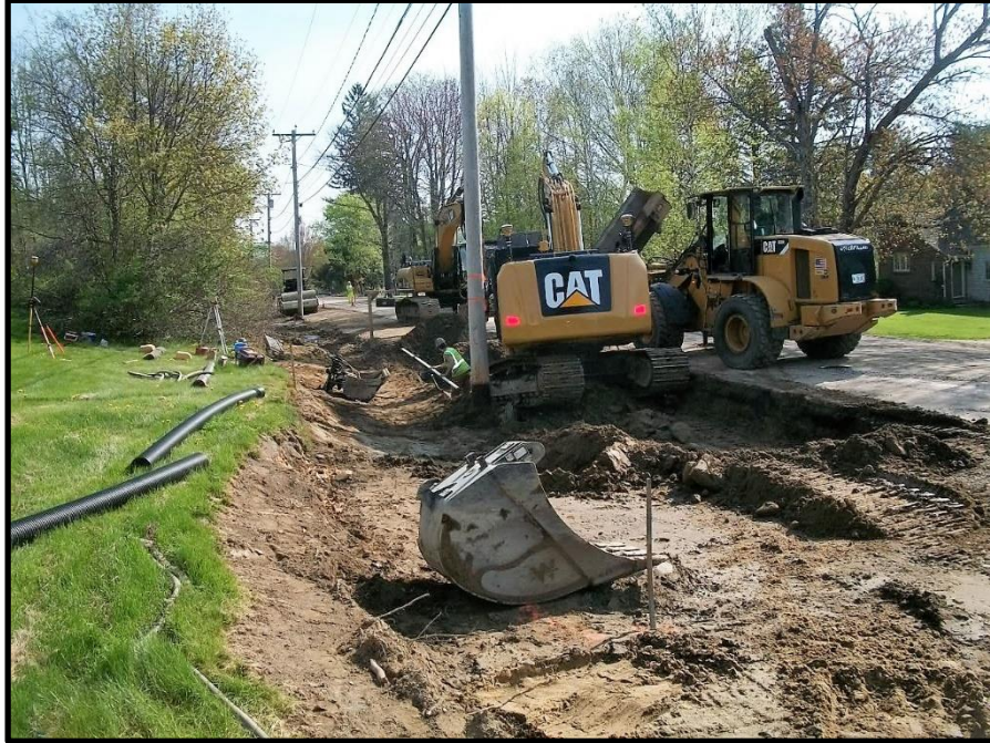
Photograph 7: Resuming the installation of 6-inch underdrain to terminate at stake in foreground at STA 68+80 in front of Butterworth Farm.
