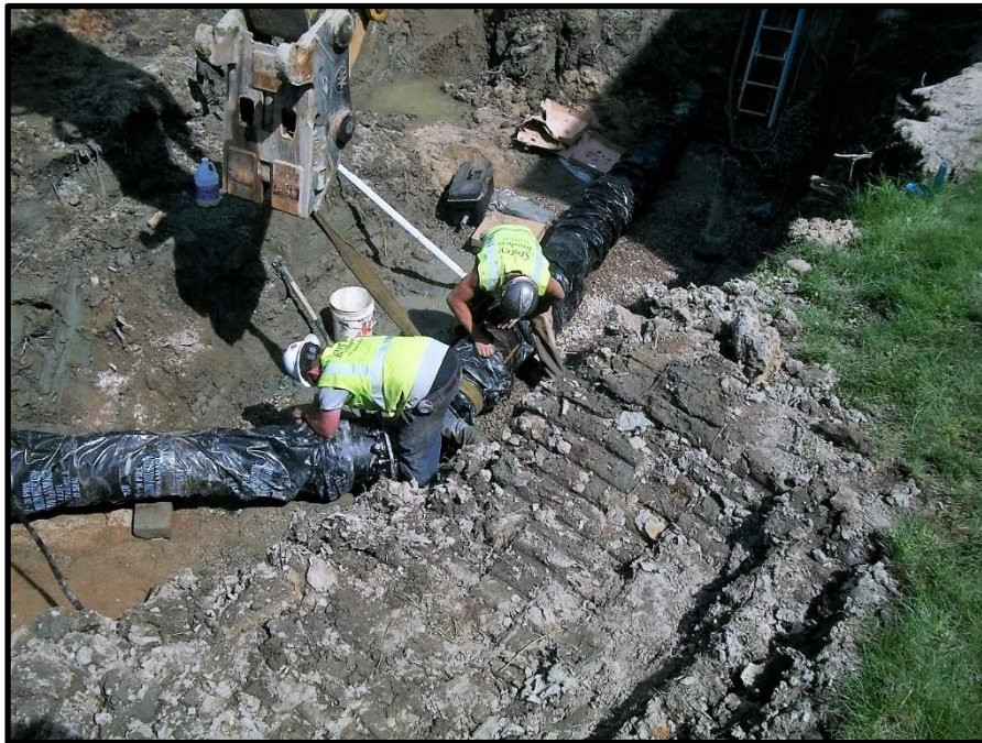
Photograph 6: Installing elbow to connect new 12-inch main from vault to the 12-inch pipe extending from the reducer pictured above.
