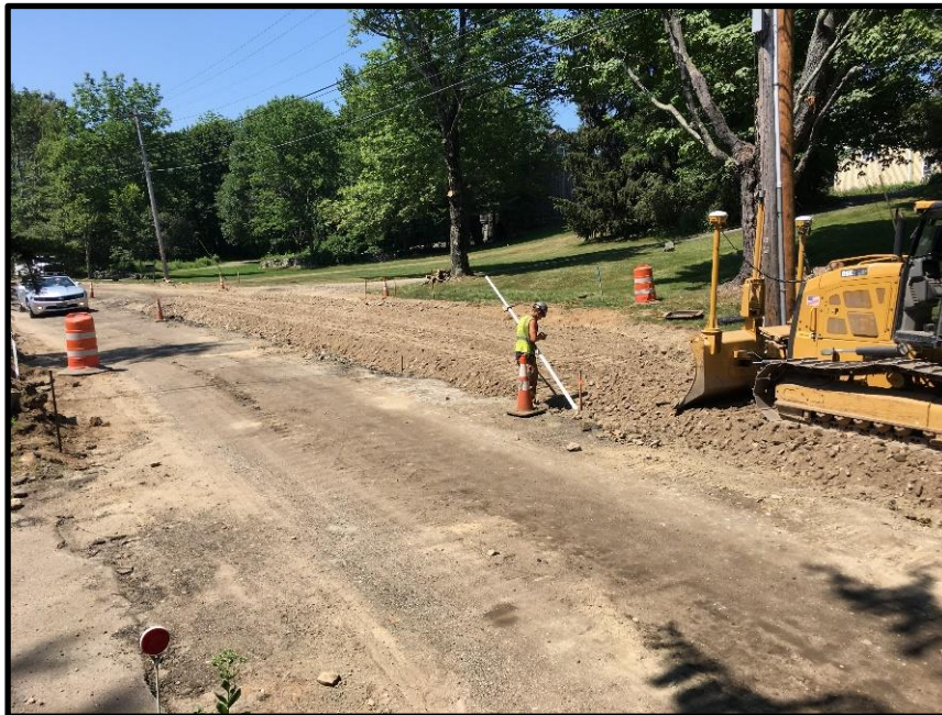
Photograph 4 - Friday, July 21 st - By late morning, crew had finished full depth reconstruction of the southbound lane to STA 49+20. Pole 318 at STA 50+03 just beyond the dozer.
