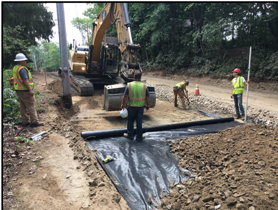
Photograph 2: Thursday, July 20 th - By afternoon, crew began full depth reconstruction of the northbound lane in a southerly direction starting from STA 52+20. Photo here taken near Pole 319 at STA 51+71.
