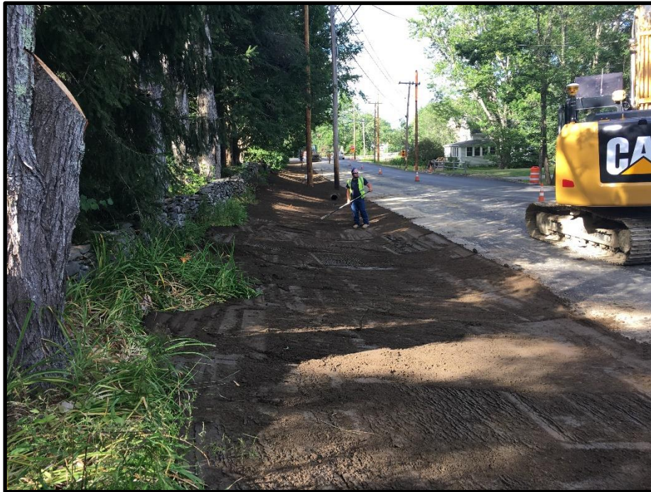
Photograph 8 - Tuesday, July 25 th - Performed preliminary finish work to previously paved section by placing loam and seed.
