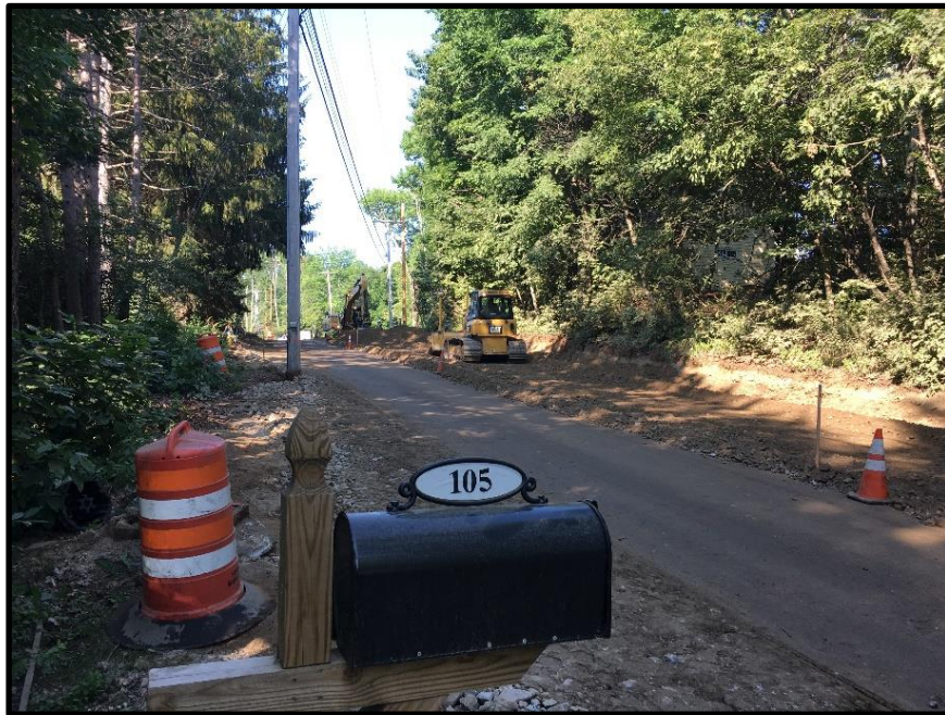
Photograph 3 – Friday, July 21 st - Began the day by resuming “full box cut” in southbound lane at STA 50+50 working south.
