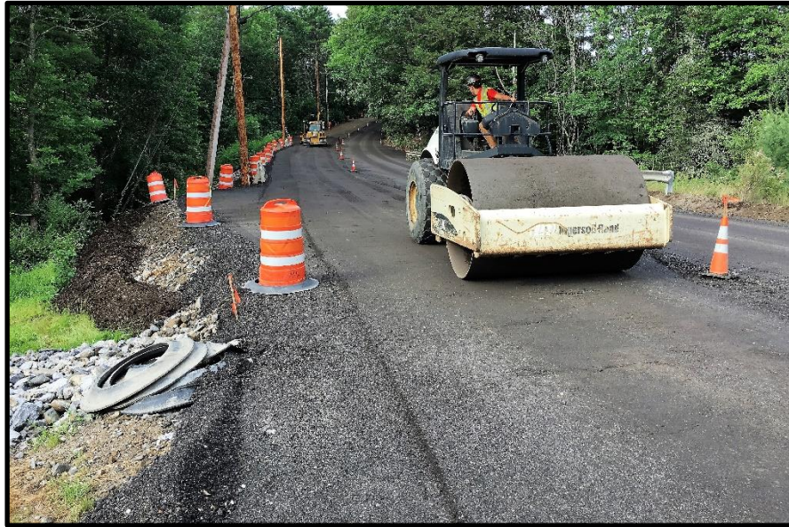
Photograph 7 – Tuesday, July 25 th - Began the day placing and compacting screened pavement millings over Type D subbase gravel in northbound lane from STA 55+80 southward to STA 48+50.
