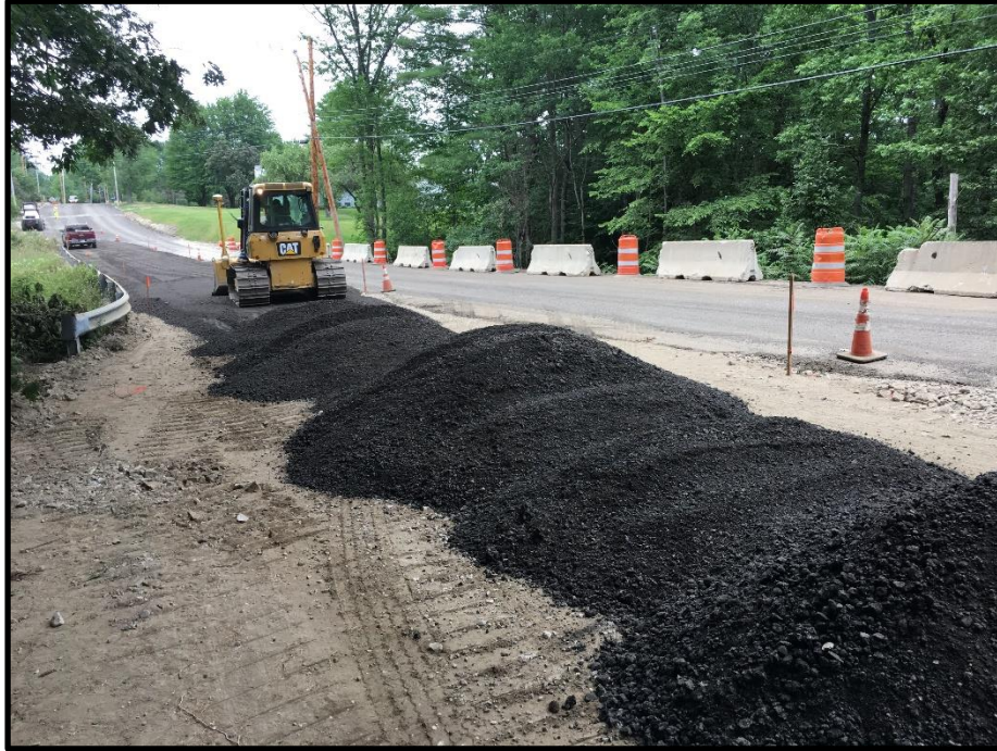
Photograph 5 – Monday, July 24 th - Began the day placing and compacting screened pavement millings over Type D subbase gravel in southbound lane from STA 57+50 southward.
