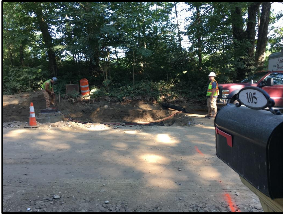
Photograph 1 – Thursday, July 20 th - Began the day by resuming “full box cut” in southbound lane at STA 52+20 working south.
