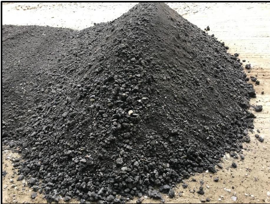
Photograph 6 - Monday, July 24 th - Close-up of screened pavement millings placed over Type D subbase gravel in lieu of Type A crushed gravel.
