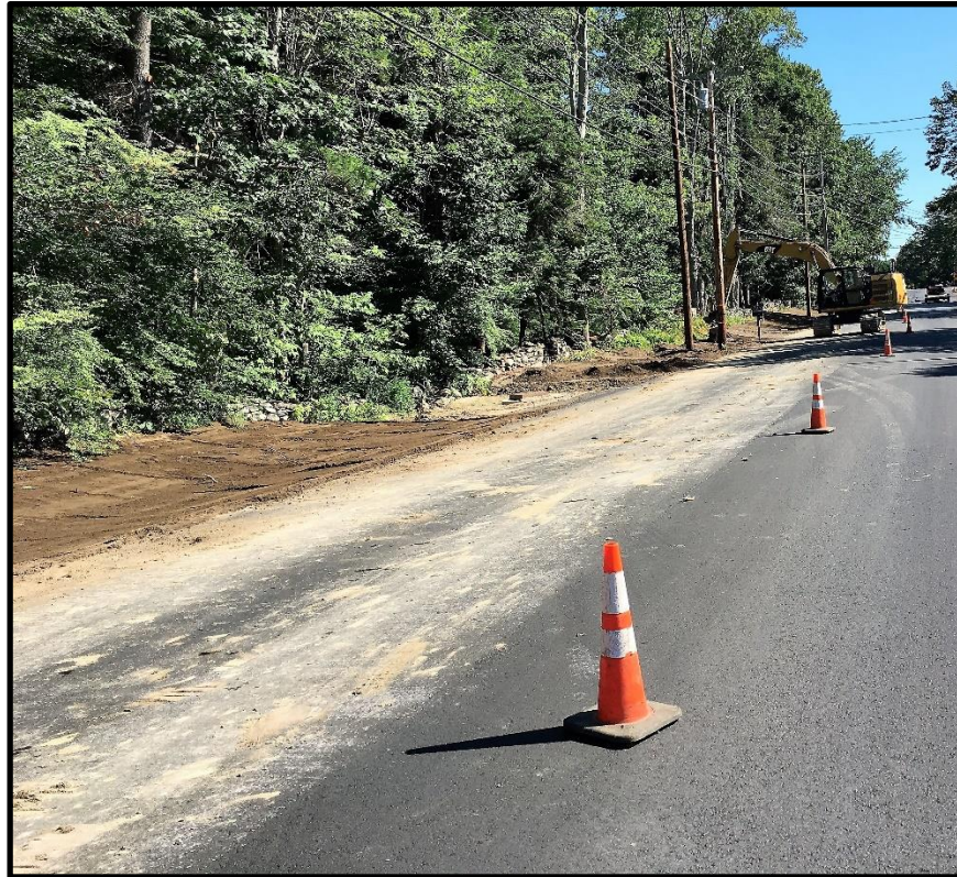
Photograph 9 – Wednesday, July 26 th – Shaping western swale prior to placing loam and seed
