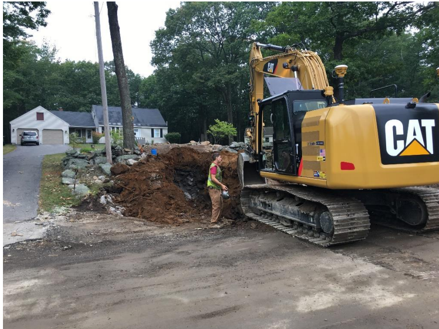
Photograph 8 - Wednesday, September 6 th - Installing “long side” water service at 70 Middle Road. Homeowner arranged with Contactor to have homeowner side blasted the previous week.
