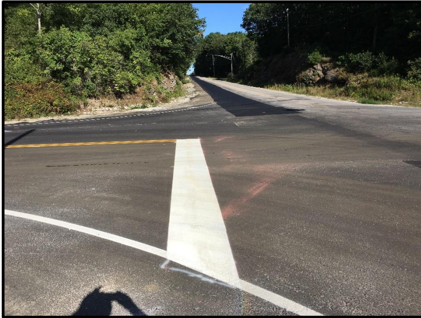
Photograph 3 – Friday, September 1 st - Installed temporary striping on paved portion of road from Tuttle Road southward to 100 Middle Road. View above is at Tuttle Road intersection looking west up Tuttle Road.
