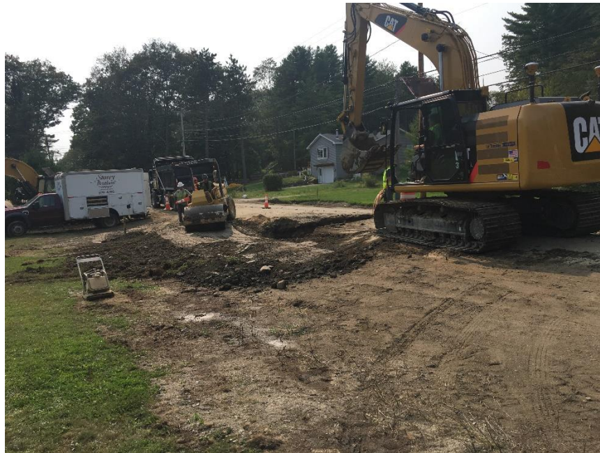
Photograph 6 - Tuesday, September 5 th - Had to use conventional open trench method when mole did not achieve proper depth.
