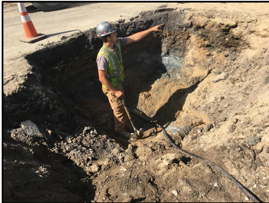
Photograph 4 - Friday, September 1 st – Using a Pneumatic Piercing Tool commonly called a “hammerhead mole” to install “long side” service under the road at 84 Middle Road to minimize traffic disruption and to avoid disturbing milled pavement.
