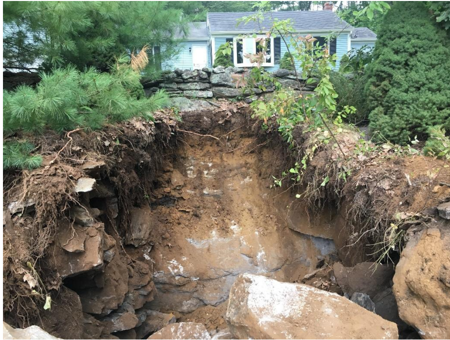
Photograph 7 – Wednesday, September 6 th - Steep ledge face at base of rock wall at 72 Middle Road. Crew to return the following day to install water service.
