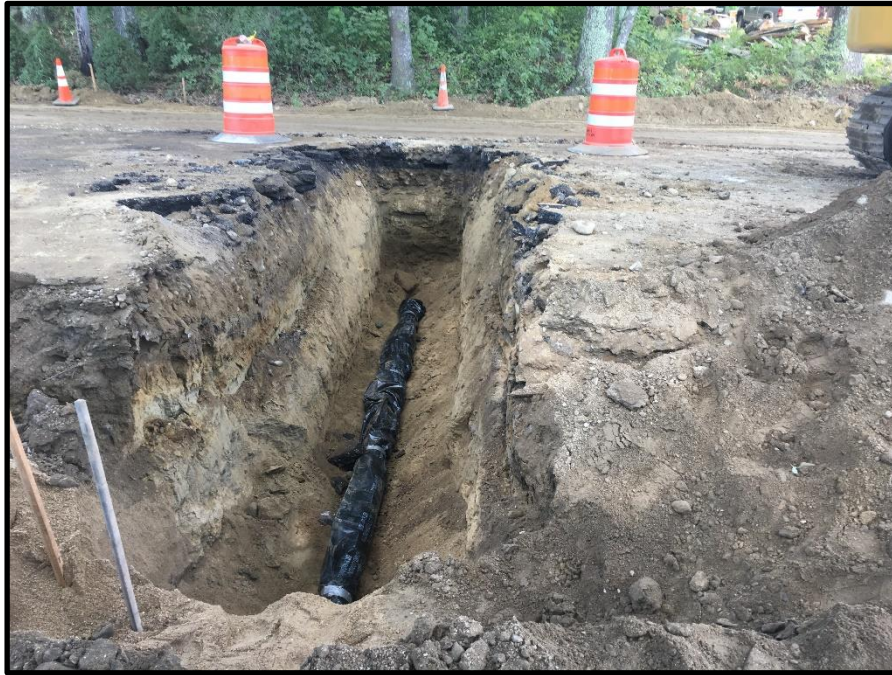
Photograph 1 – Thursday, August 31 st - Trenching across road for hydrant at 76 Middle Road (STA 37+60).
