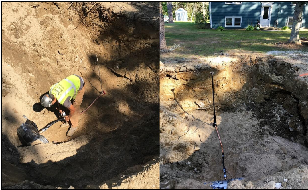
Photograph 2: Thursday, August 31 st – Installing new water service from new water main extension at 77 Middle Road at location preferred by the homeowner for convenient connection later.
