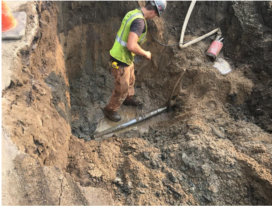
Photograph 5 – Tuesday, September 5 th – “Long side” services were mainly installed via the “Pneumatic Mole.” Copper service line was pulled through the void which helped minimize traffic disruptions.
