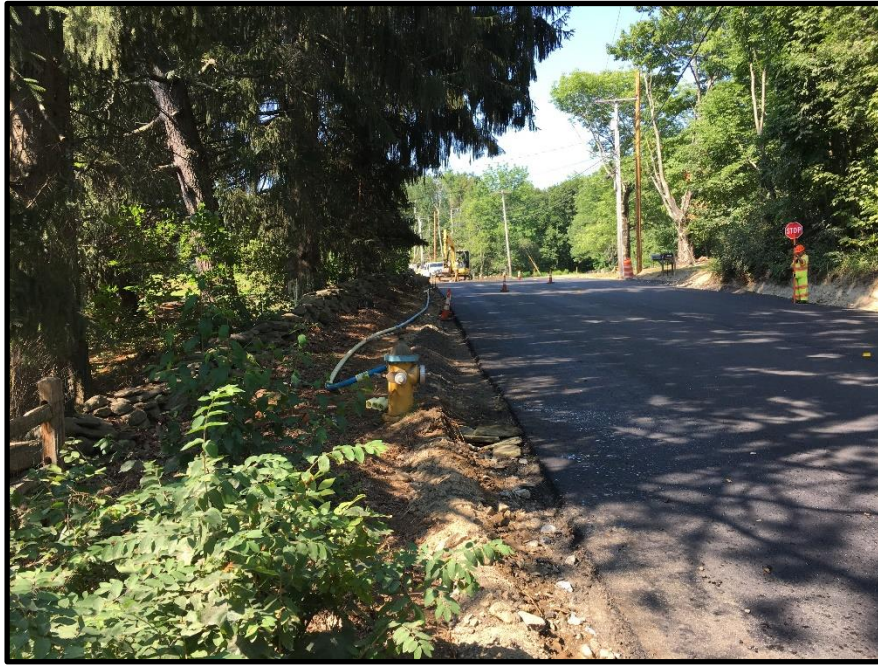
Photograph 7 – Tuesday, August 1 st - Started day installing temporary water main from hydrant (at STA 51+21, RT) extending 350 feet southward to serve houses #95, #97, #99, & #100.
