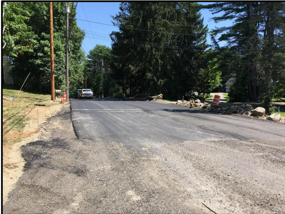
Photograph 6 - Monday, July 31 st - Southern terminus of pavement after 2nd layer of base pavement was placed in the northbound lane of the current work zone.
