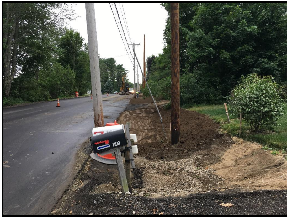
Photograph 1 – Thursday, July 27 th - Freshly loamed and seeded swale north of 142 Middle Road (looking north).
