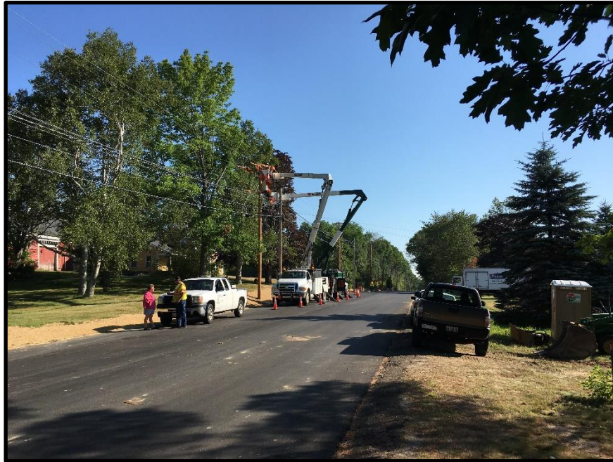
Photograph 9 – Wednesday, August 2 nd – On Target Utility Services started day transferring CMP wires near Butterworth Farm Road north of Storey Brothers loam work.
