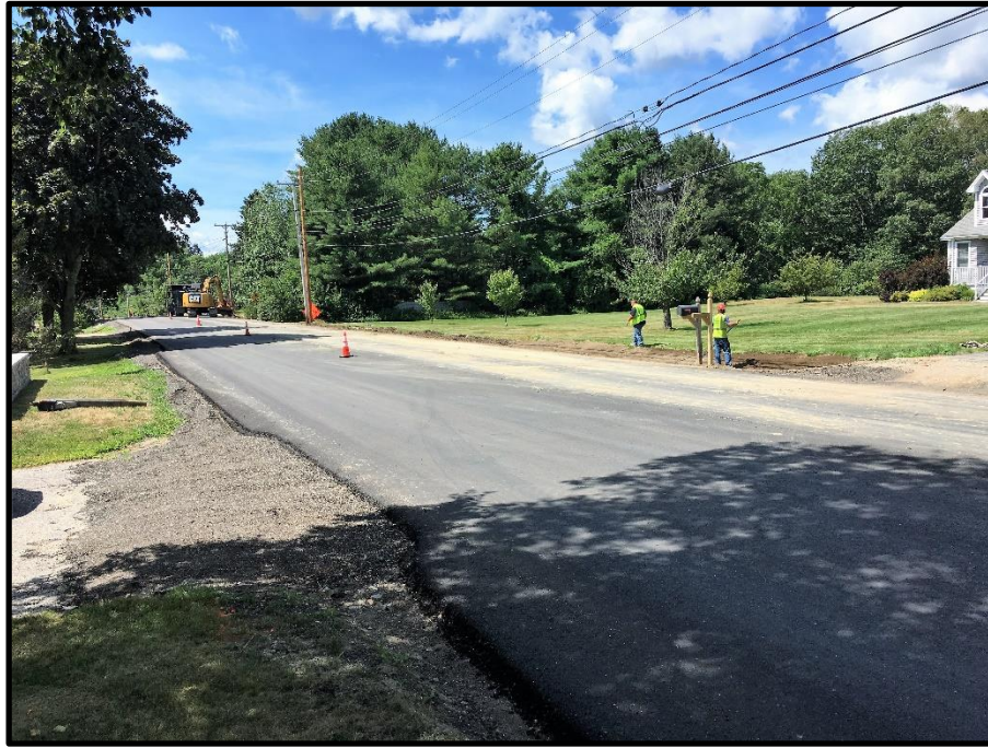
Photograph 3 – Friday, July 28 th - Shaping swale and placing loam southerly from Butterworth Farm Road along the west side of road in front of 126 Middle Road.
