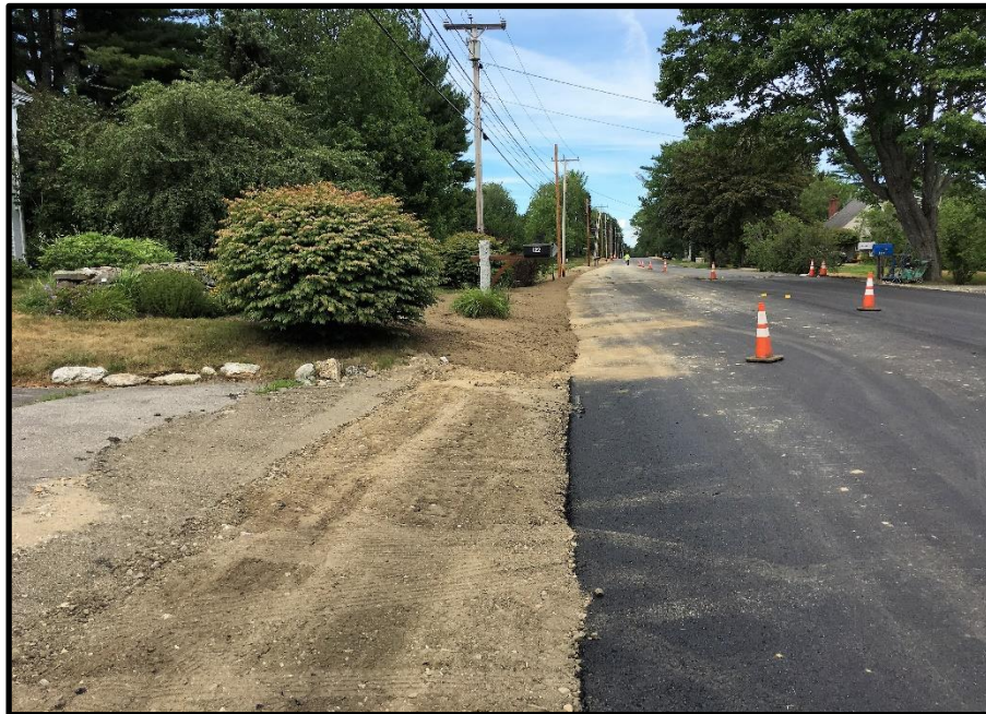
Photograph 4 - Friday, July 28 th - Southern extent of loam & seed at STA 61+10 (Eddy driveway at 122 Middle Road) prior to the placement of straw mulch at the end of the day.
