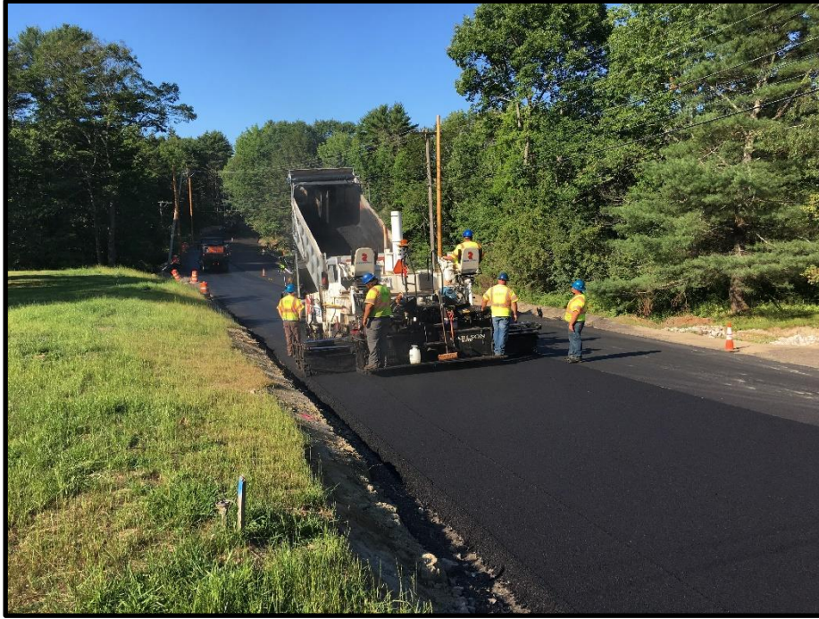
Photograph 5 – Monday, July 31 st - Crew from Glidden Paving just underway at 8AM placing 2nd layer of base pavement.
