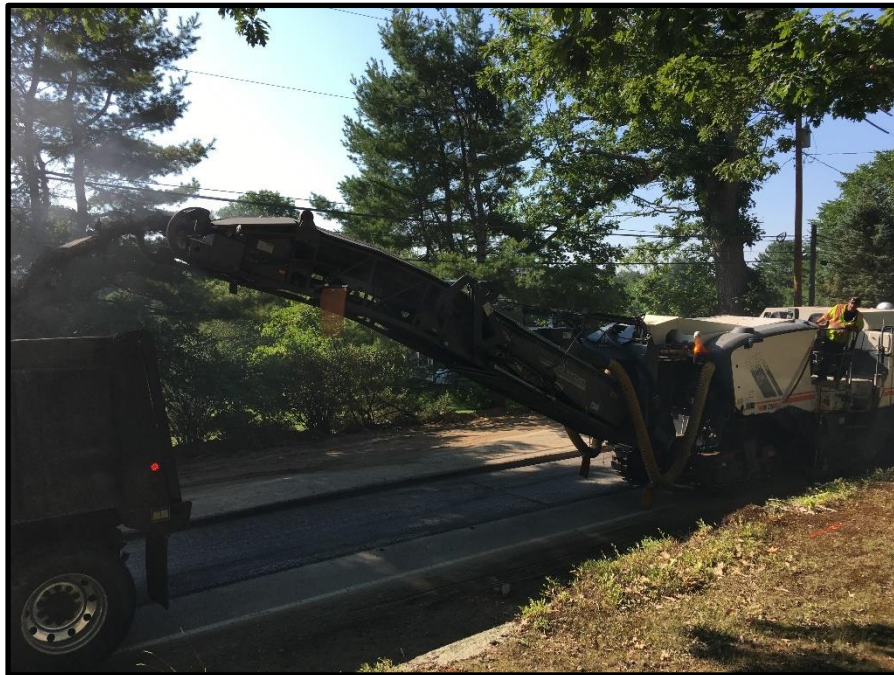
Photograph 2: Thursday, August 10 th - Milling shoulder of southbound lane in a northerly direction and conveying the millings onto trucks. These millings will be used later on the road as the top layer of gravel.
