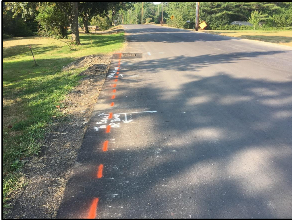
Photograph 9 – Wednesday, August 16 th – Layout for placement of bituminous curb to be installed later in the day by J. Parsons Paving.
