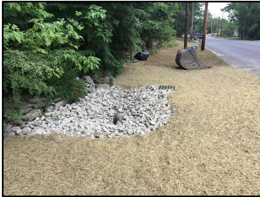
Photograph 7 – Tuesday, August 15 th - Installed a field inlet to the underdrain inlet pipe of CB-7E to pick up flow from an intermittent stream west of the rock wall. This catch basin had to be raised so outlet could clear water main.
