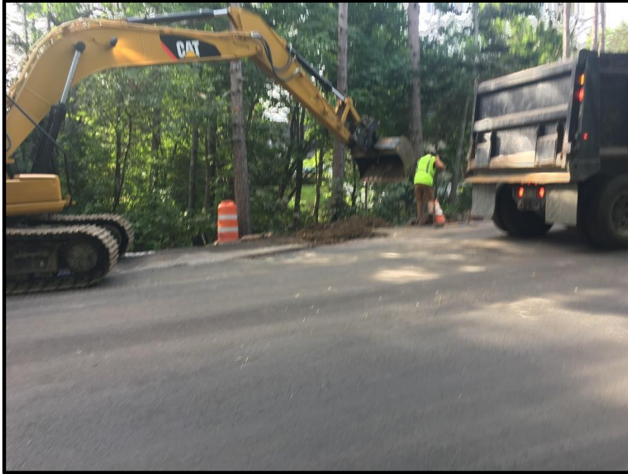
Photograph 5 – Monday, August 14 th - Saw cut around existing catch basin structures that were paved over in the gully section and then excavated to expose them to install frame & grate to new grade. Shown here is the existing catch basin at STA 52+00, Right.
