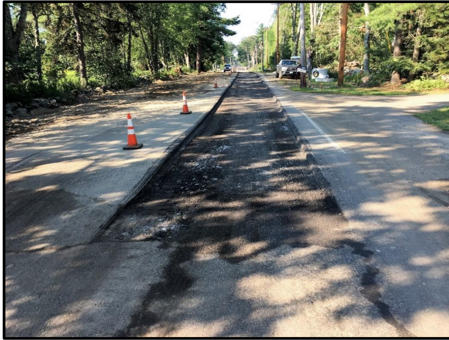
Photograph 1 – Thursday, August 10 th - Beginning of 8'2' wide x 3 ½ inch deep pavement milling in southbound travel lane at STA 49+50 (near 95 middle Road) looking southward.
