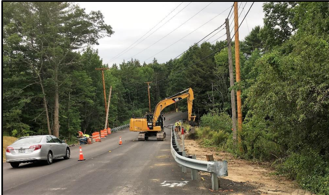
Photograph 8 - Tuesday, August 15 th - Removed the old guard rail on the inlet side of the Chenery Brook culvert. Cleared away weeds & small brush and leveled ground behind guardrail. Afterwards, placed loam, seed, & mulch.
