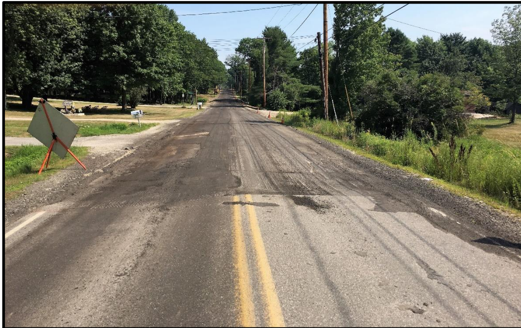
Photograph 4 - Friday, August 11 th - A view looking north from southern end of pavement (near 50 Middle Road) that was milled yesterday by Coastal Road Repair.
