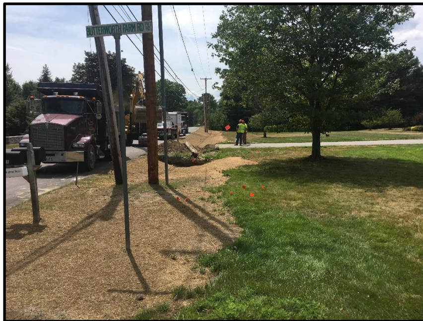
Photograph 6 - Monday, August 14 th - Installed new driveway culverts north of gully. Driveway for 126 Middle Road shown here at STA 65+00, Left.
