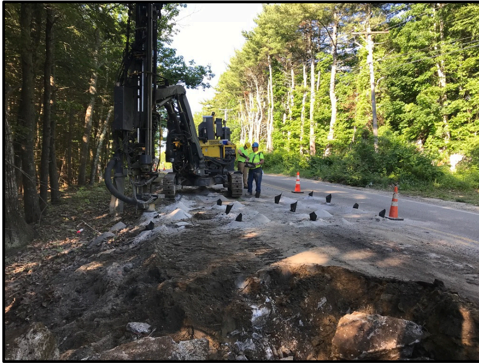
Photograph 7 – Wednesday, June 20 th – Drilling for first blast of the day
