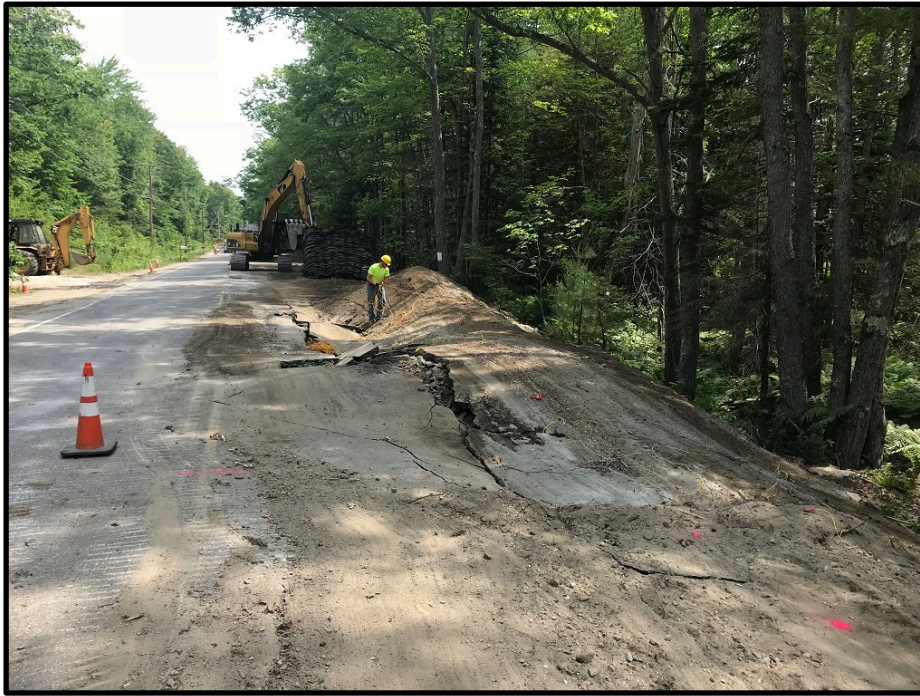
Photograph 5 – Monday, June 18 th – Removing blasting mats after a blast
