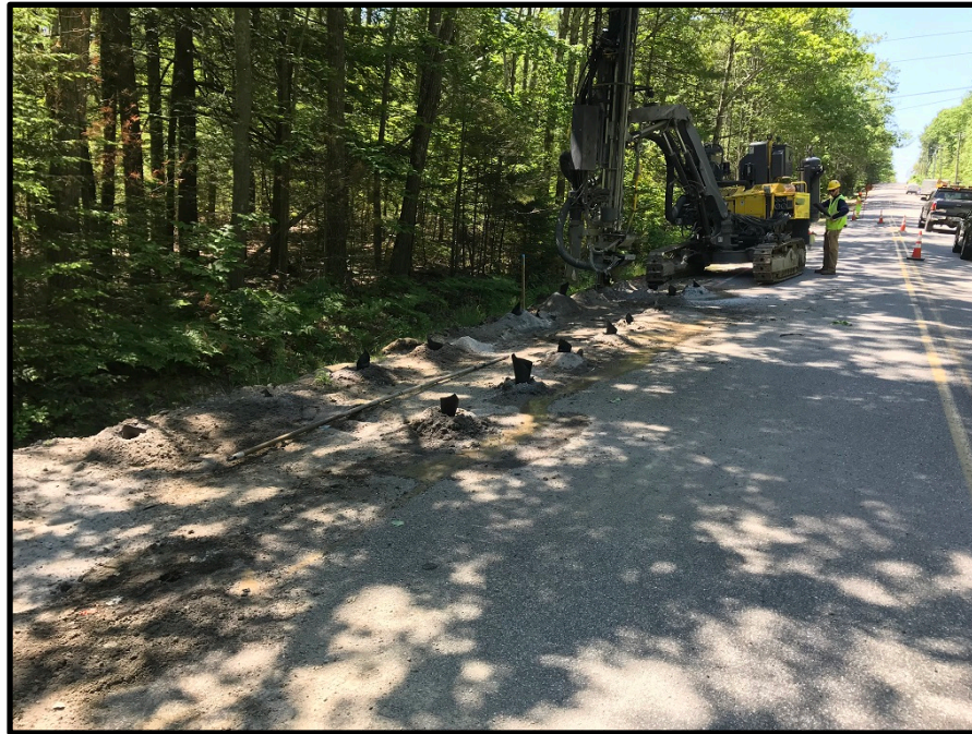
Photograph 3 - Monday , June 11th – Drilling for blasting bedrock just north of Evergreen Lane
