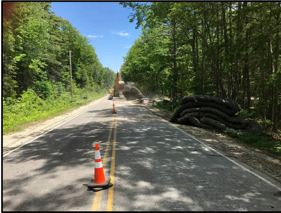
Photograph 7 – Wednesday, June 13 th – Placing blasting mats
