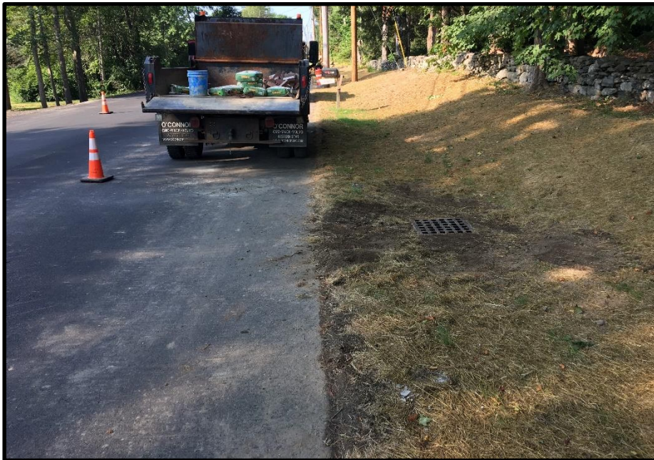
Photograph 6 - Monday, August 7 th - Storey Brothers installed frame & grates on catch basins and prepared driveways for pavement from Tuttle Road southward. CB-8B shown here.
