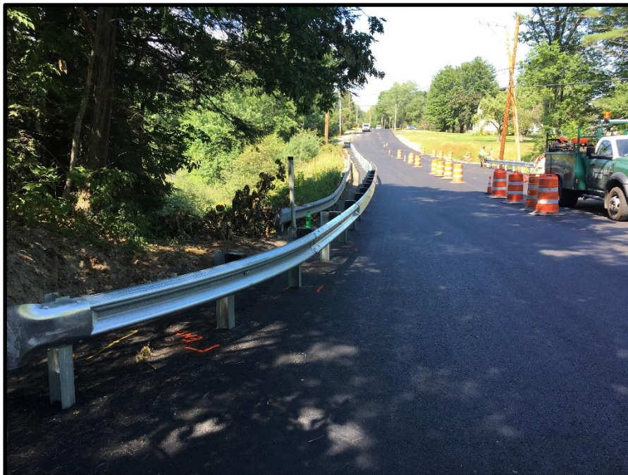
Photograph 2: Thursday, August 3 rd - North of blasting operation, Maine Line Fence installed guard rail on west side of Chernery Brook Gully then set up to install on east side before relocating to install guard rail on the east side of road from 153 to 157 Middle Road.
