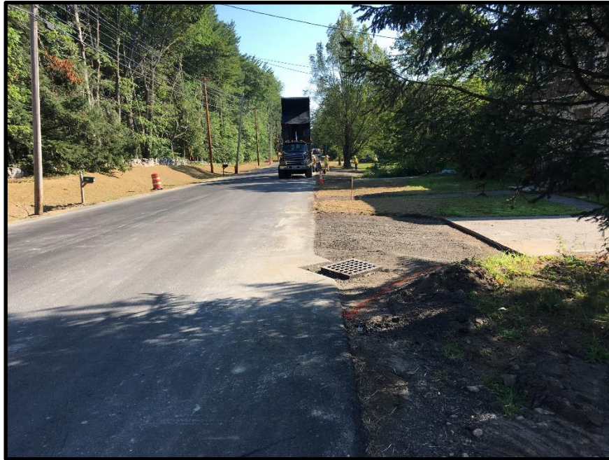
Photograph 9 – Wednesday, August 9 th – Driveway apron for 147 Middle Road prepared for paving. Paving crew in background placing pavement at 151 Middle Road driveway. Catch Basin CB-7D in foreground.
