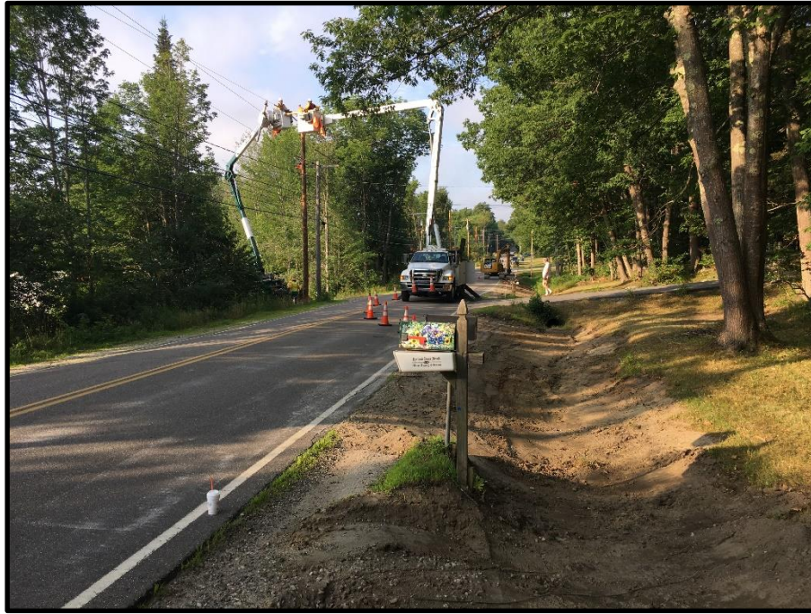
Photograph 3 – Friday, August 4 th - On Target Utility Services started day transferring CMP wires just south of Range Way and north of Storey Brothers grubbing and excavating for drainage along the shoulder.
