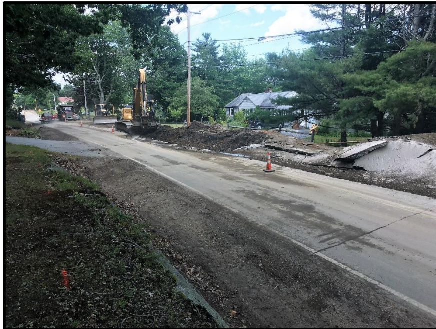
Photograph 10 - Wednesday, August 9 th - Storey Brothers supports blasting operation by removing broken pavement and lifted soil after blasting prior to grading with dozer and compacting with roller to re-establish the travel lane for traffic.
