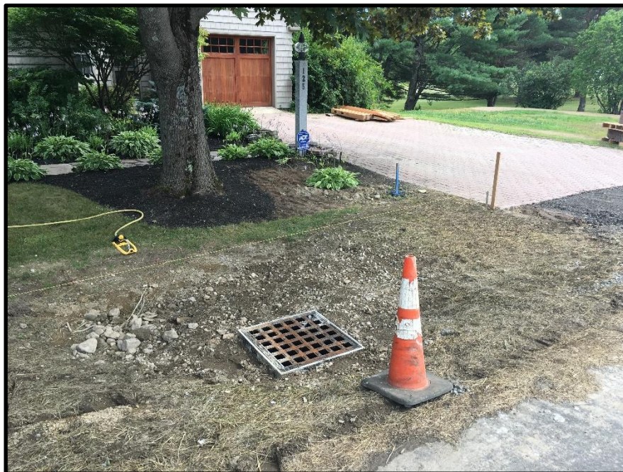
Photograph 8 - Tuesday, August 8 th - Storey Brothers installed frame & grates on catch basins and prepared driveways for pavement. CB-6E shown here in front of 125 Middle Road prior to placing loam & seed.
