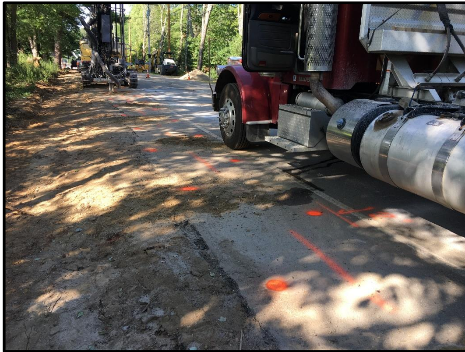
Photograph 1 – Thursday, August 3 rd - McGoldrick started drilling and blasting ledge for water main extension trench from STA 48+00 southward marking overburn depths every 10 feet.
