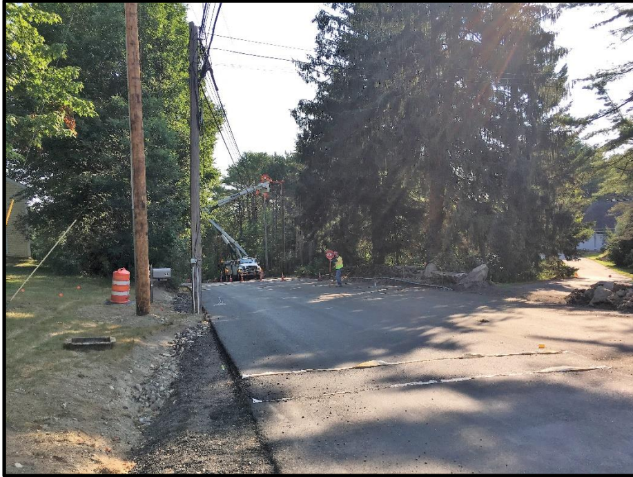
Photograph 5 – Monday, August 7 th - View looking north of On Target Utility Services transferring CMP wires on replacement Pole #319 just south of the Chernery Brook Gully in front of 101 Middle Road.
