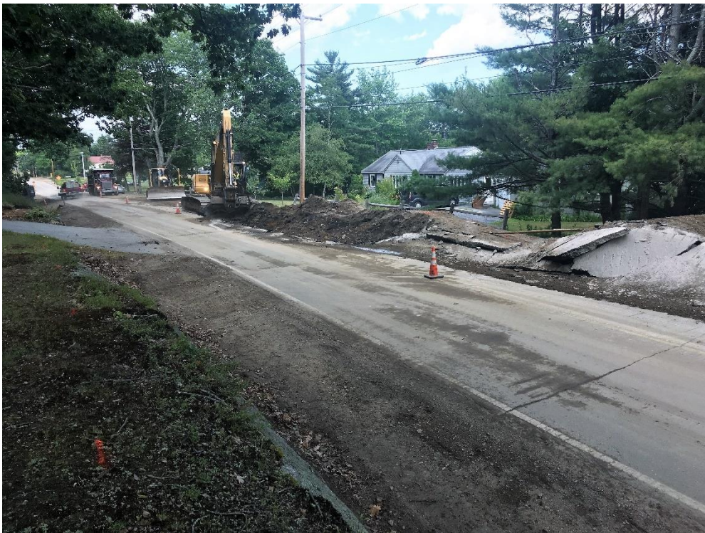
Storey Brothers removing broken pavement and lifted soil from blasting prior to grading with dozer and compacting with roller to re-establish the travel lane for traffic.
