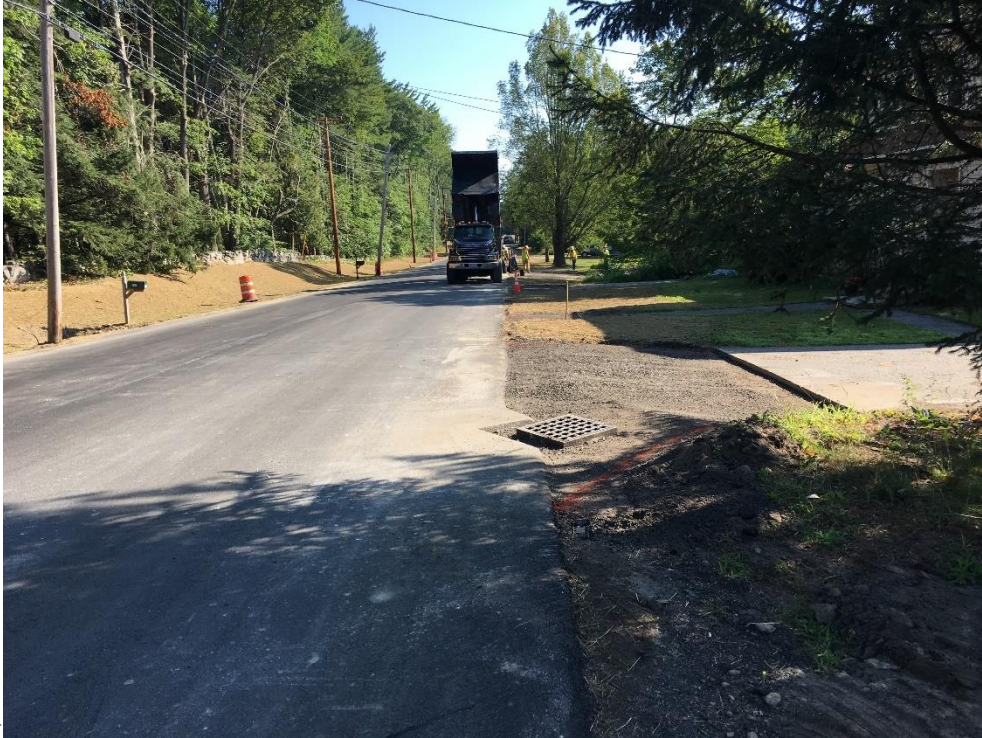
Driveway apron for 147 Middle Road prepared for paving. Paving crew in background placing pavement at 151 Middle Road driveway.
