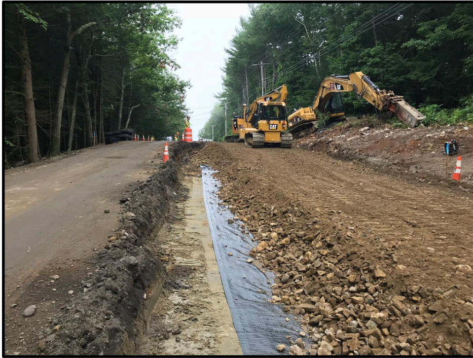
Photograph 7 – Tuesday, July 24 th – Grading subbase gravel between 10 and 4 Middle Road
