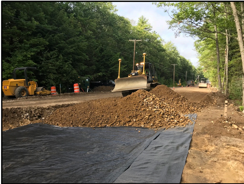
Photograph 6 - Monday, July 23 th – Placing subbase gravel
