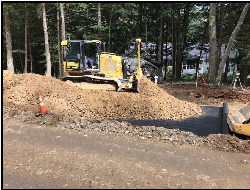
Photograph 8 - Wednesday, July 25 th – Placing subbase gravel near Tall Pines Way
