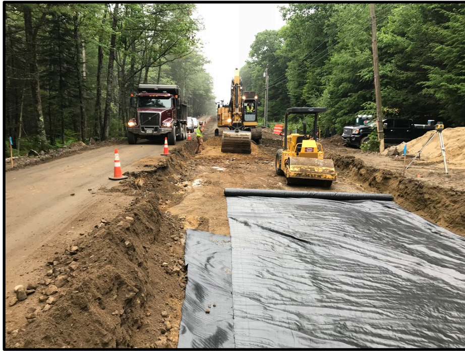
Photograph 5 – Monday, July 23 th – Excavating to base grade near existing bus turnaround
