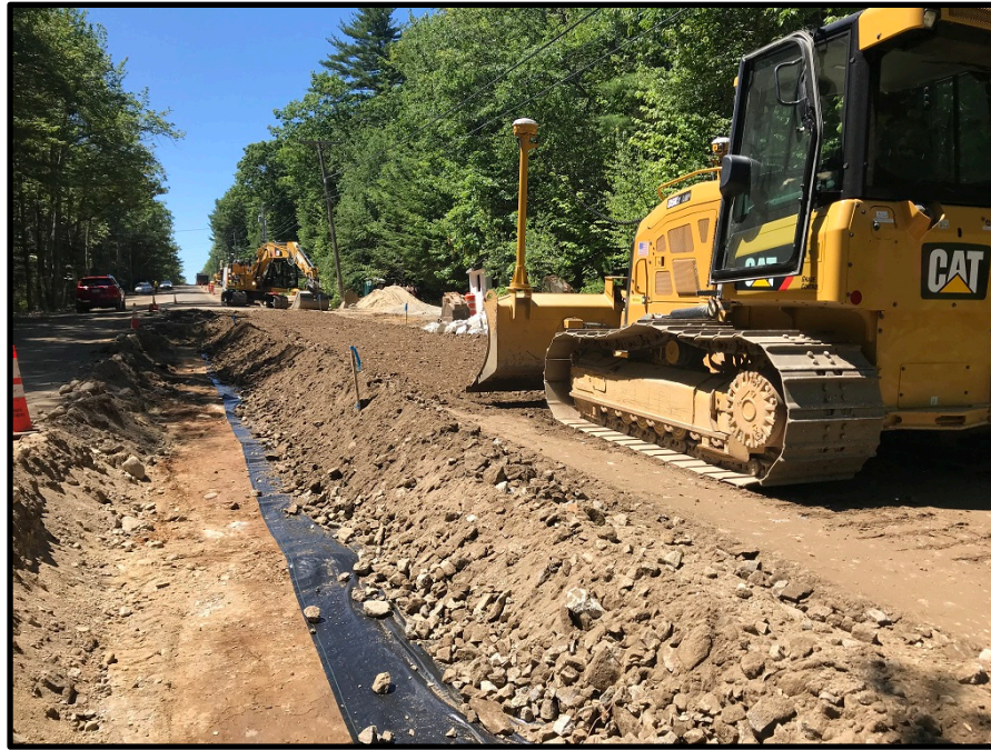
Photograph 3 - Friday , July 20 th – Grading subbase gravel near existing bus turnaround
