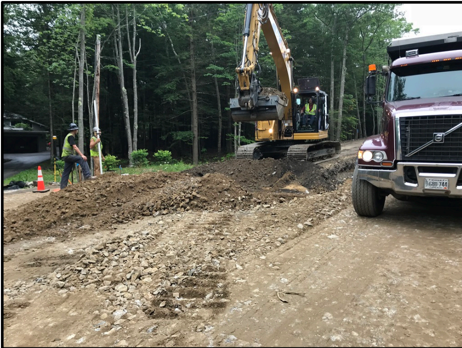
Photograph 8 - Tuesday, July 24 th – Excavating for base grade near 15 Middle Road
