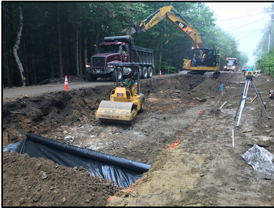
Photograph 7 – Wednesday, July 25 th – Excavating for base grade near Tall Pines Way
