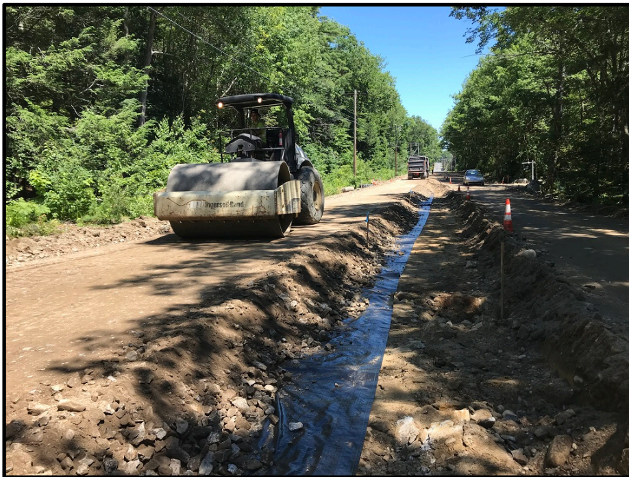
Photograph 4 - Friday, July 20 th – Compacting subbase gravel
