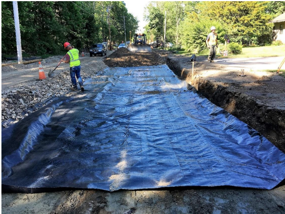
Near the end of the day on east side of road. View shows exposed subgrade with geotextile fabric in foreground and dozer placement of new gravel in background.
