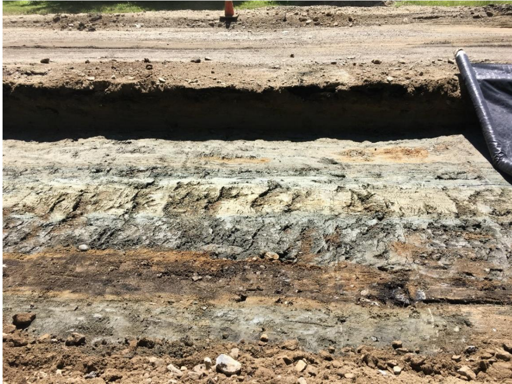
Morning excavation to subgrade of road at STA 77+50 (across the street from 153 Middle Road) with soft clay in foreground and firmer clay in background.
